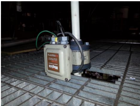
Figure 3.11. System Slurry Flowmeter.
