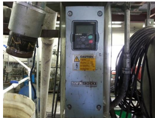
Figure 3.10. PLC Motor Controller.
