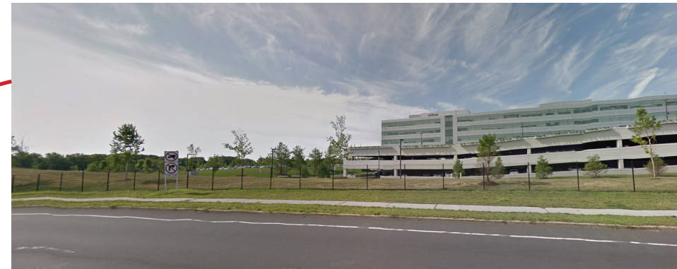
Street view from S Service Rd
