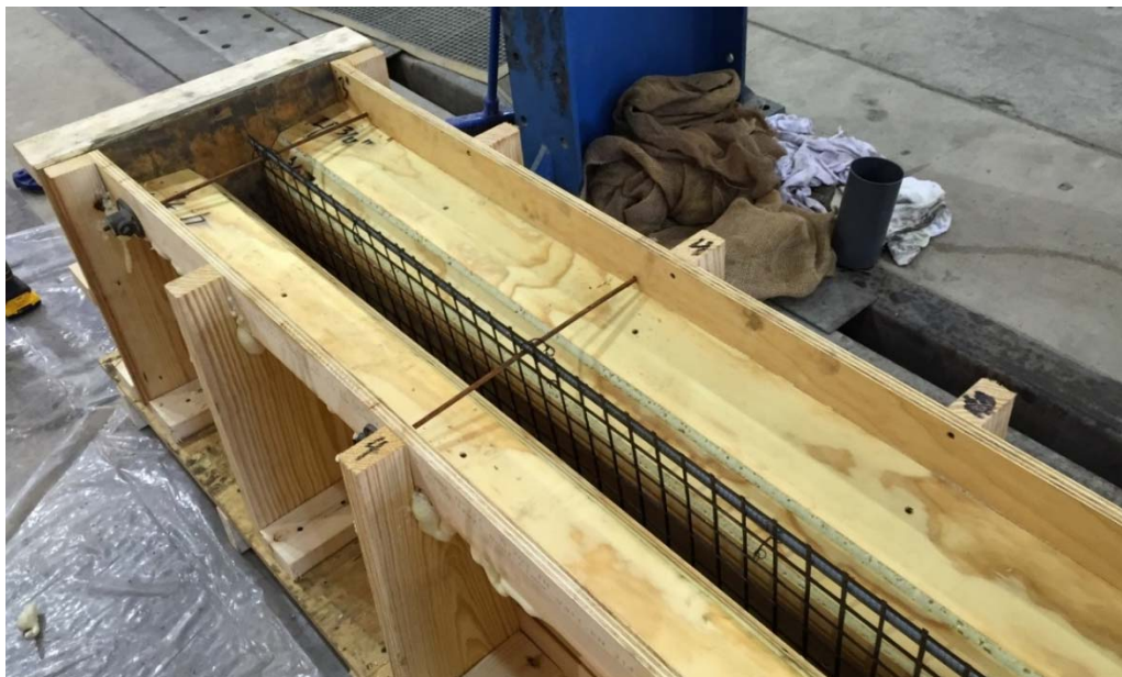
Figure 18: Completed Beam Formwork with C-Grid
