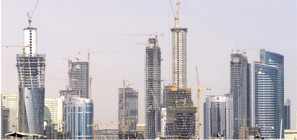
Figure 1.1: Tall buildings under construction in Doha, Qatar (QNRF 2015)
