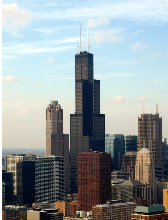
Figure 1.2: Chicago’s Willis Tower is an example of a bundled tube (Gerometta)
