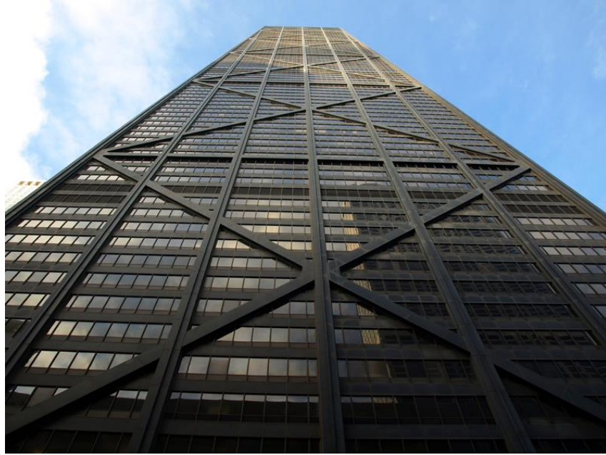
Figure 1.3: Chicago's John Hancock Center employs a trussed tube design (Gerometta)
