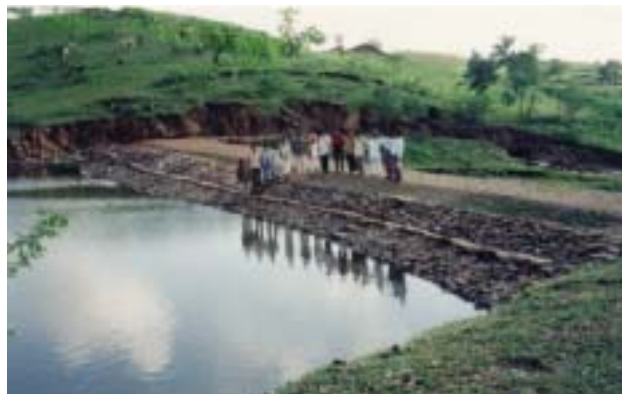
PLATE 21 Detention of sediment-laden runoff by a dam wall has been used to provide limited areas of flat cropland (here under rice); this may have been one of the purposes of the dam. Sharam, India [T.F. Shaxson]
