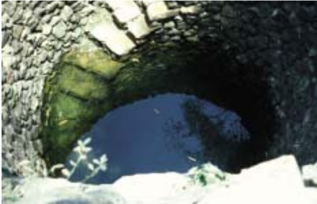
PLATE 23 Dug wells such as this one may go dry because the water table falls below the depth to which the well was dug. Palampur, India [T.F. Shaxson]
