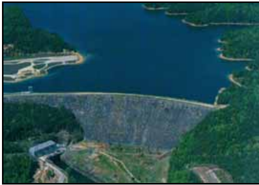
The 300-foot tall Lewis Smith Dam is one of the largest earth and rock-filled dams in the eastern United States
