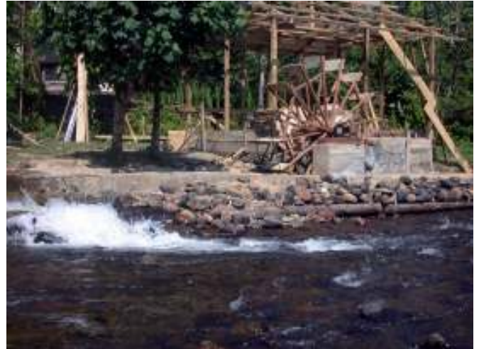
Construction of small-scale hydropower facility that allows villagers to get electricity from their stream proved to be an incentive to maintain the forested landscape mosaic intact, with its global benefits
