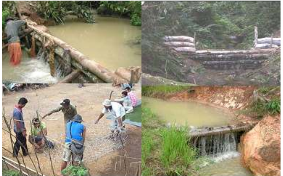
RiverCare: interventions to stabilize river channel and reduce sediment loads
