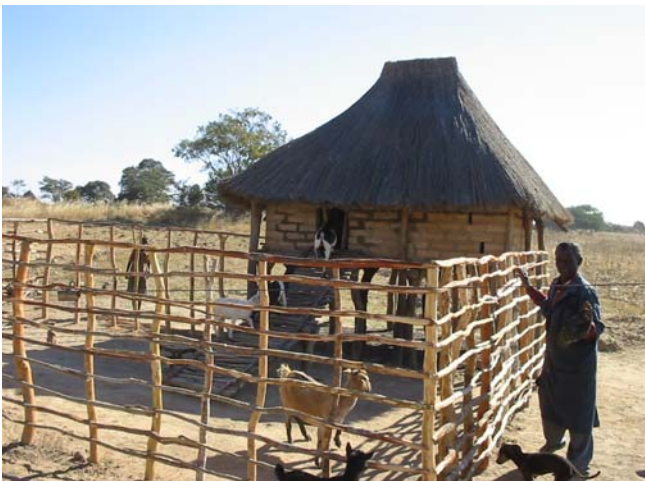
Figure 3 - Example of a stand-alone shelter that uses less trees than an all wood shelter. Note the spaces left between bricks for ventilation. Photo courtesy of Heifer Project International, Zambia.
