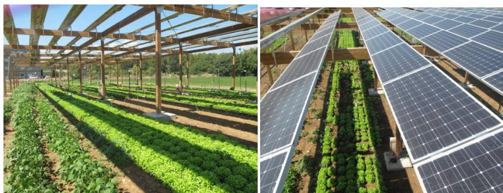
Figure 10 : A prototype of an agri-voltaic system combining solar panels and field crops. A 4 m clearance allows easy mechanization of the system with conventional machinery. Location : Montpellier, France
