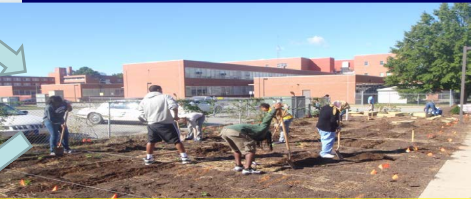
Students transporting & leveling soil
