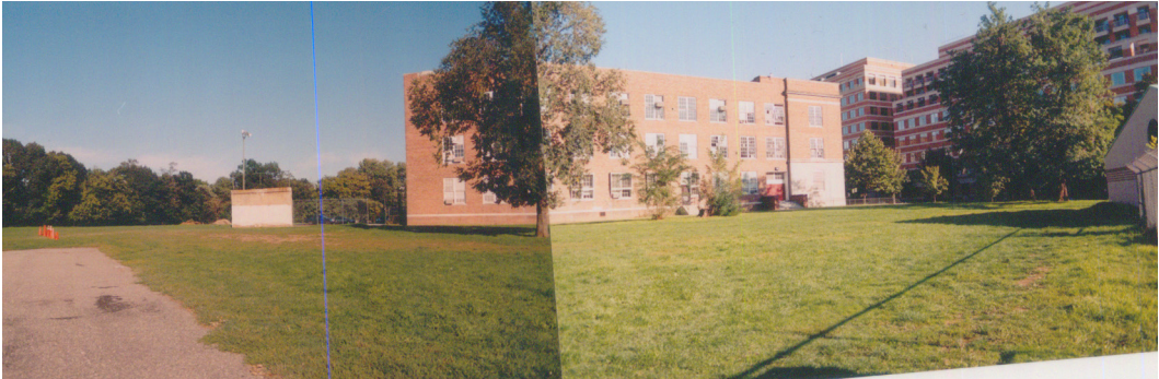
Site, Looking Northwest
