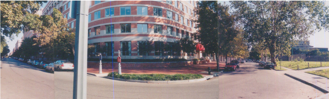
Site, Adjacent Office Building
