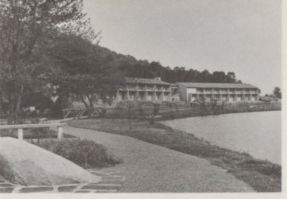
PEAKS OF OTTER LODGE, MILE 85.6 After crossing the James River, the parkway ascends 3,286 feet in 13 miles to its highest elevation in Virginia, 3,950 feet.
