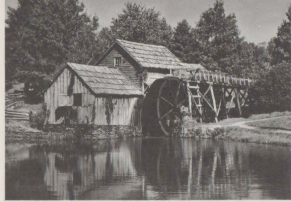
MABRY MILL, MILE 176.1 Blue Ridge Parkway passes through a region rich in the folk history of the late 1700's, when the Blue Ridge marked the edge of the western frontier. Log cabins, farm buildings, a church, and a gristmill are some the structures preserved as evidences of the pioneer past.
