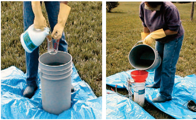
Figure 1. Determine the amount of chlorine bleach or calcium hypochlorite needed, mix, and pour the chlorine solution into the well. Source: Minnesota Department of Health. www.health.state.mn.us/divs/eh/wells/waterquality/disinfection.pdf .
