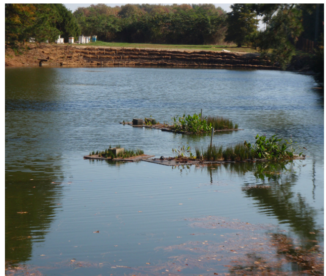
Figure 3. Floating treatment wetland (FTW) rafts in a pond located at Virginia Tech's Hampton Roads Agricultural Research and Extension Center in Virginia Beach, Va.
