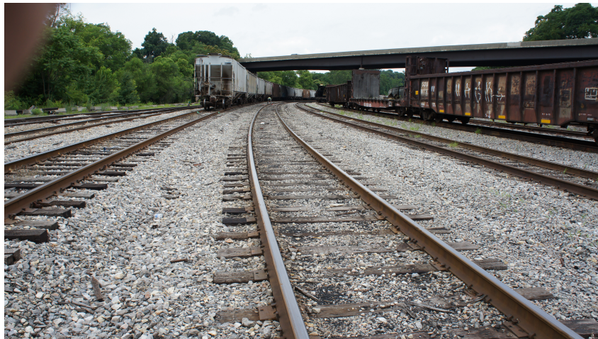
Figure 3-1 Yard curved section of track
