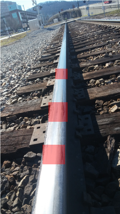
Figure 6-10 Section of the rail after the lubricator showing discrete patches of lubricant
