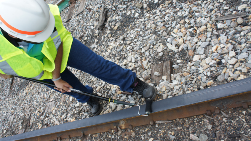
Figure 3-5 Applying TOR lubricants using small roller
