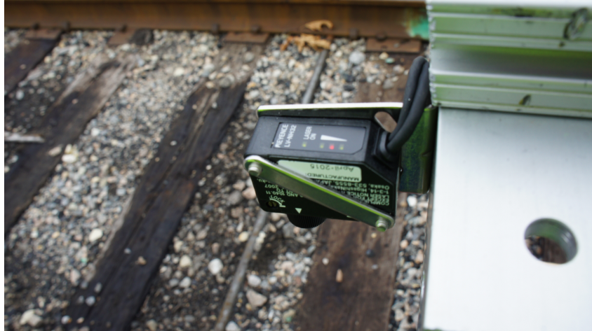
Figure 3-2 Laser head mounted 3 ft. high with respect to rail
