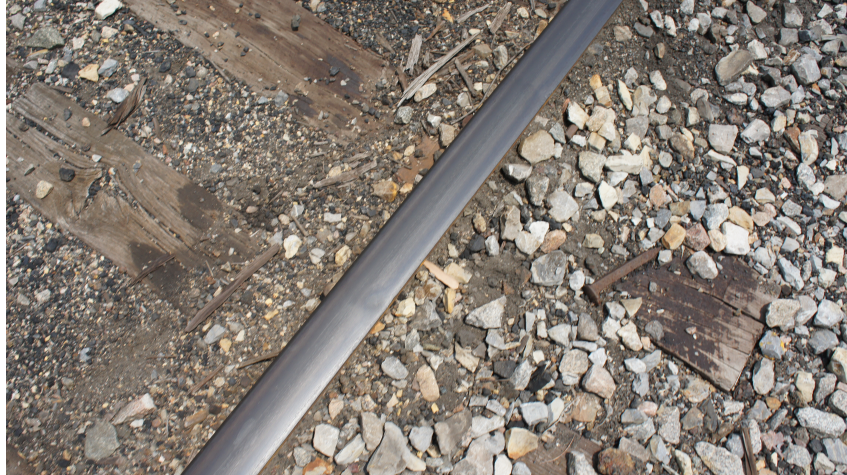
Figure 3-6 A thin layer of Lubricant C on top of rail
