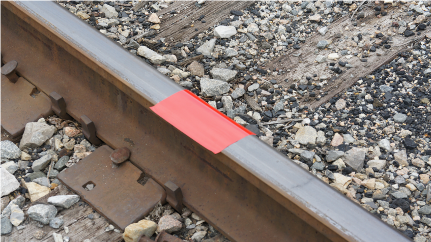
Figure 3-4 Red reflective tape acts as rail sections markers
