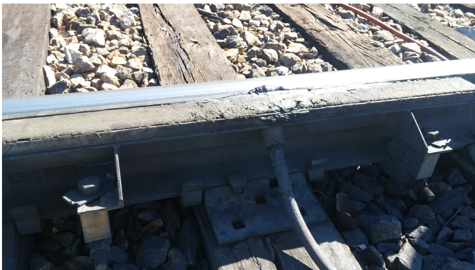
Figure 6-3 Close-up picture of the lubricator pumping lubricant on top of rail
