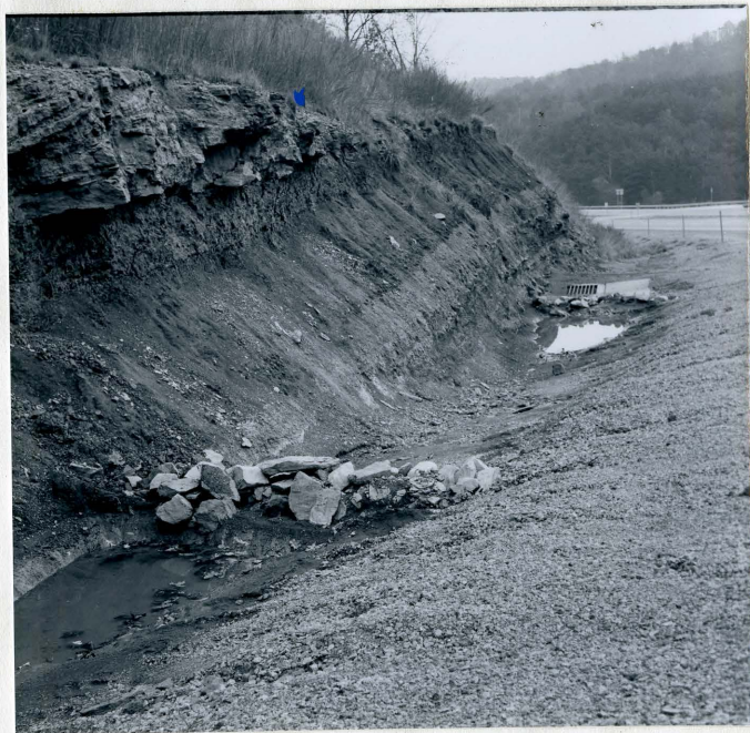
Figure 3. Top: Bench grading with broad benches to catch falling materials creates very steep back slopes, making it difficult to obtain protective vegetation. Bottom: Erosion and sedimentation into ditches are serious problems. Sediment dams were made with rocks, to reduce clogging of drains and culverts.
