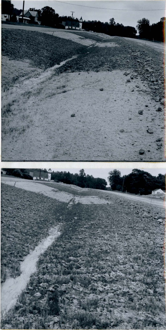
Figure 10. Top: Foreground shows conventional smooth hard grading with little vegetation; background shows rough, loose tillage with vigorous seedlings. Bottom: A closeup of the roughened, cloddy subsoil shows excellent stands and growth of seedlings 21 days after seeding.
