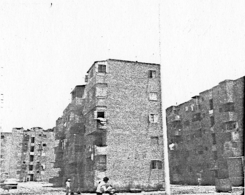
Figure 24. Disparities in the housing situation in Cairo.
