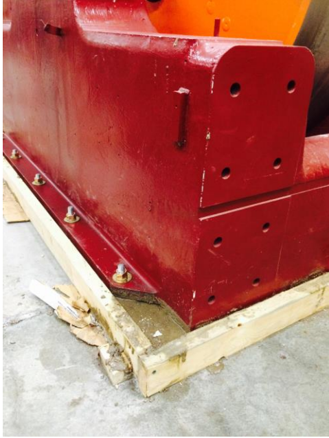
Figure 23: Grouting of the Machine
