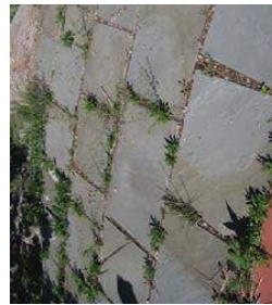
Weeds ready to be removed in cracks between pavers in a gathering area.
