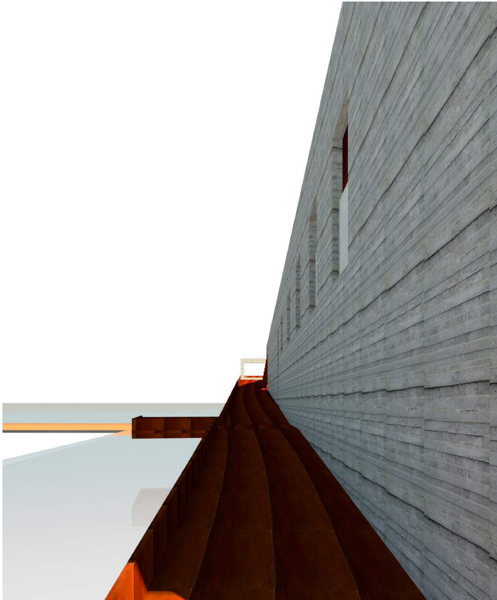
View of the ramp at the entrance. The exterior walls are of board formed finished concrete. The flooring and railing of the ramp are of corten steel.
