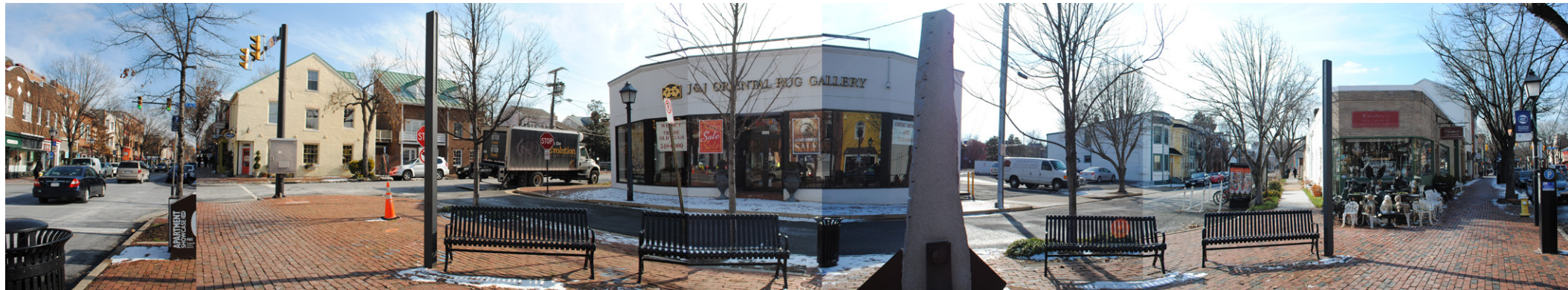
Panoramic Photo of Existing Building and Site
