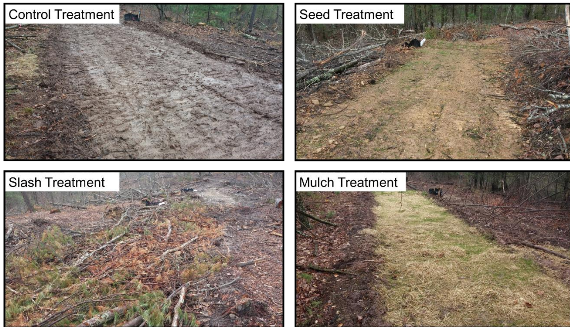
Figure 2.3: Comparison photographs of each BMP treatment following project installation. Note the downslope waterbar with sediment trap in each photo.
