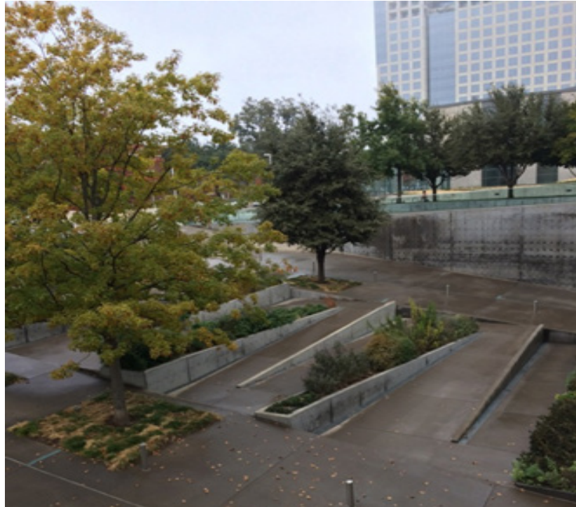
Figure 6- Zigzag entry ramp system to the Dee and Charles Wyly Theatre, Dallas, Texas. Original Photo by the Author
