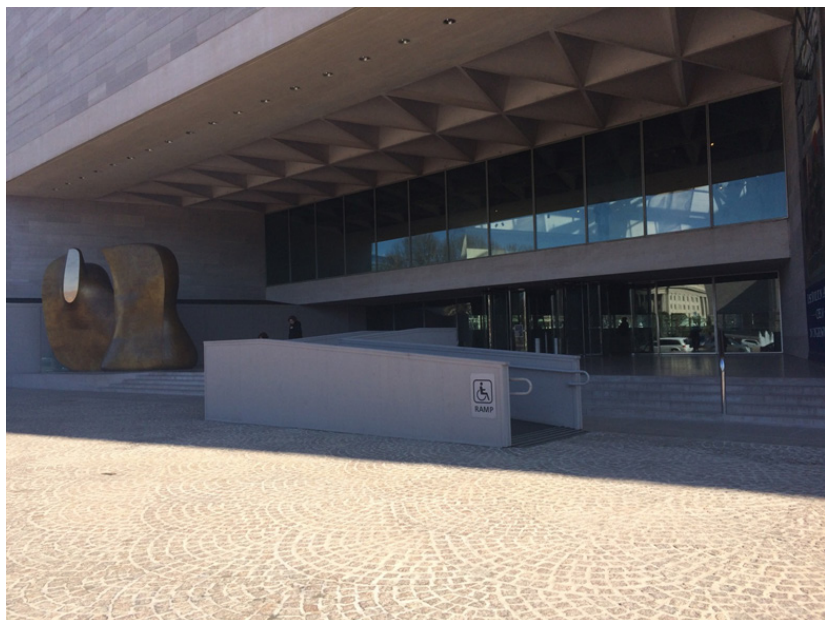
Figure 12 – National Gallery of Art East Wing, Washington, DC entrance. This image shows the addition of a ramp to the entry staircase. Original Photo by the Author
