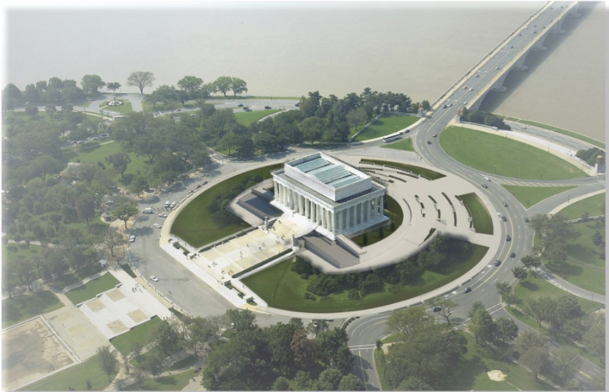
Figure 38 – Aerial Photograph of The Lincoln Memorial including the western newly designed entrance.
