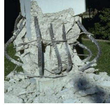
(c) Hoop rupture (1979 Imperial Valley earthquake).
