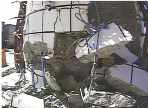
(a) Cover spalling
