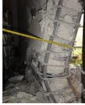
(b) Out-of-plane buckling (2011 Christchurch earthquake).
