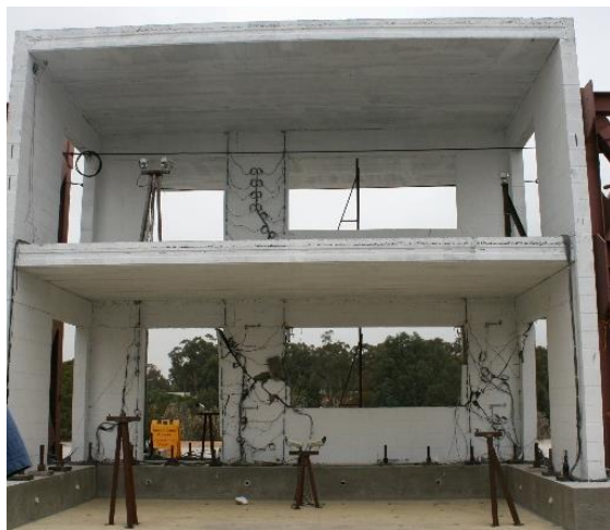
(a) Crack patterns at the end of the experiment
