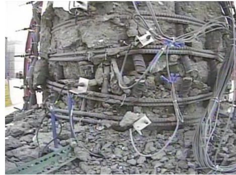
(b) Rebar buckling, concrete crushing and subsequent rebar rupture
