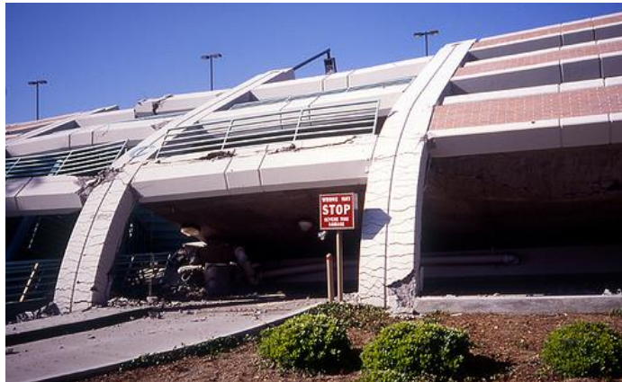
Figure 1.1: Ductile collapse of a 4-story parking garage at California State University (Northridge Earthquake 1994).
