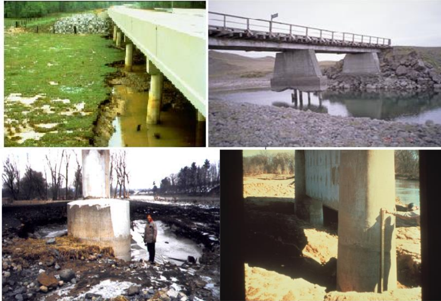
Figure 1. Bridge failures due to local scour (adopted from USGS).
