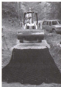
In Virginia, Best Management Practices can help minimize sedimentation resulting from forestry operations. Practices include the use of temporary bridges (left) and geowebbing (right) for stream crossings during logging operations. Photos by: Mike Aust, Virginia Tech.
