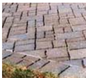
Dry Laid Pavers
