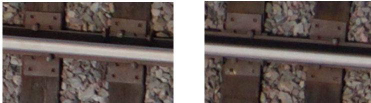
Figure 6.1: Images from El Paso Sub Division [36]
