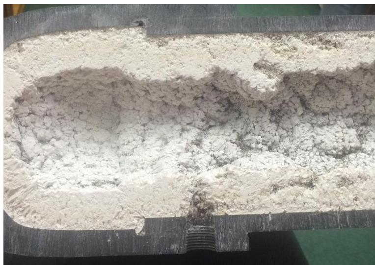
Figure 8 - Struvite Buildup at HRSD's Nansemond WTP in Suffolk, VA
