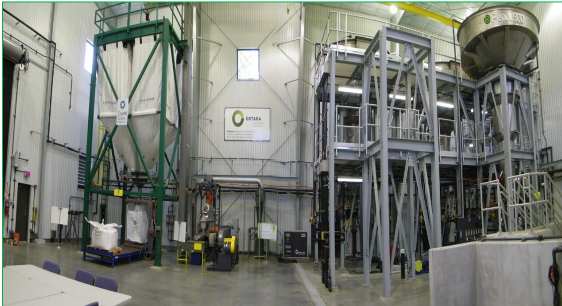
Figure 2 – Ostara Nutrient Recovery Technologies Inc. Struvite Recovery Facility at HRSD's Nansemond WWTP in Suffolk, VA
