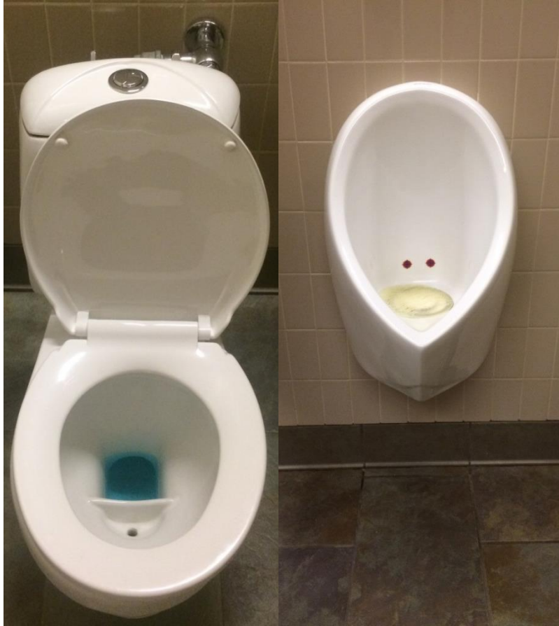
Figure 12 - Urine-Separating Toilet & Waterless Urinal at HRSD's Main Office in Virginia Beach, VA
