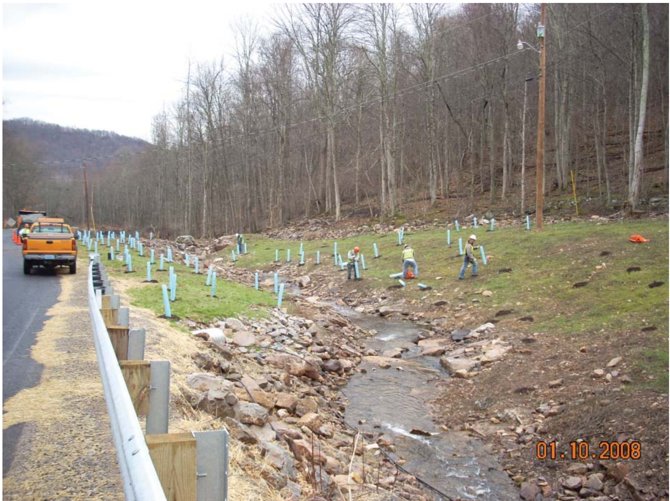
Little Stoney Creek realignment example in Giles County, Virginia. Photo courtesy of Justin Laughlin, DGIF
