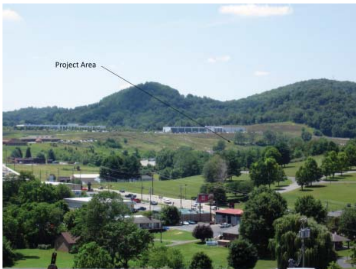
Photo of project site taken from the Russell County School Board offices.
