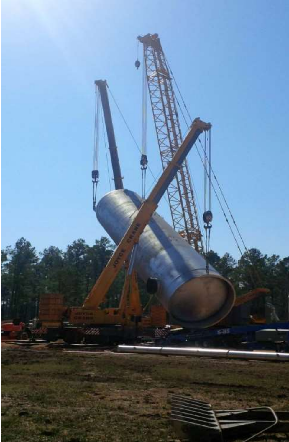
Figure 54: Lifting the World's Largest Contained Burn Structure into Place 545
