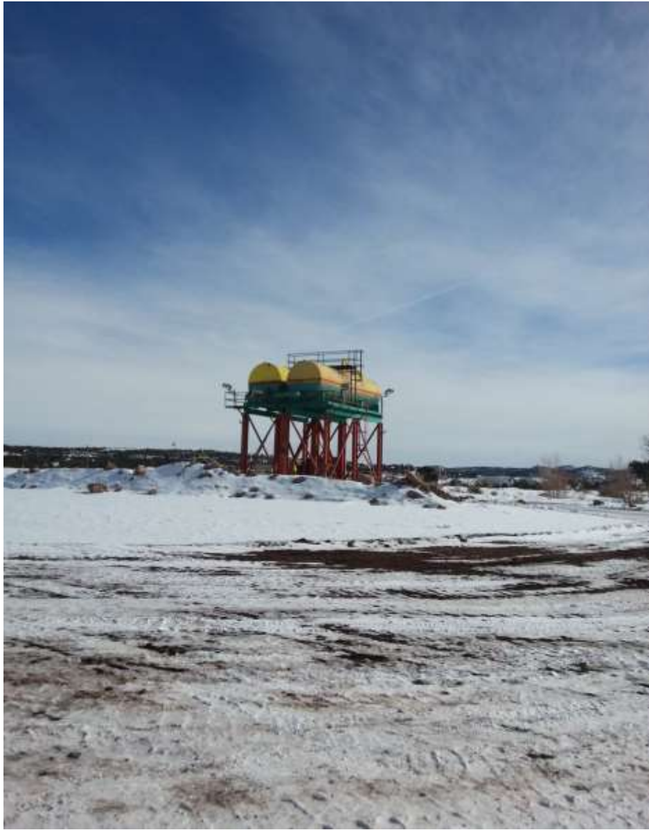
Figure 27: Chemical Storage Tanks
