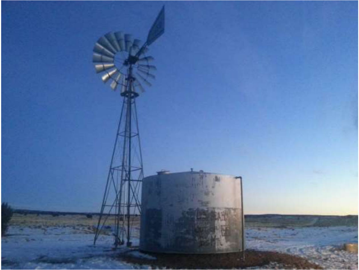
Figure 7: Water Well on the Fenceline
