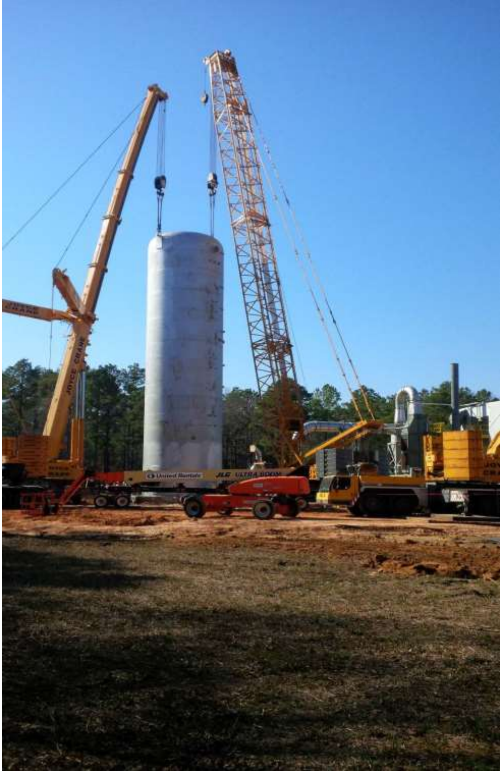
Figure 55: The World's Largest Contained Burn Chamber in Place 546
