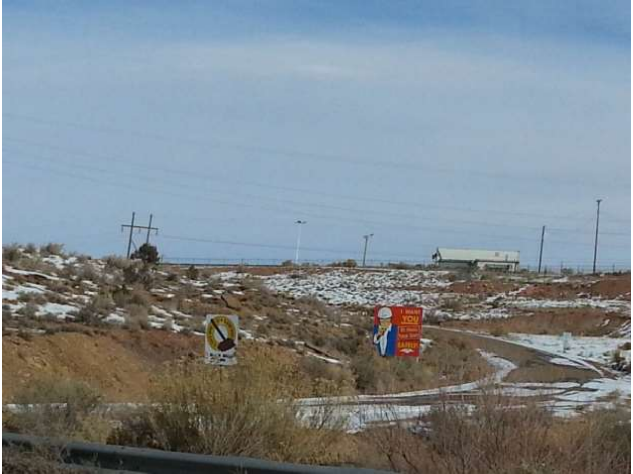
Figure 6: Entering the Slurry Complex at Black Mesa
