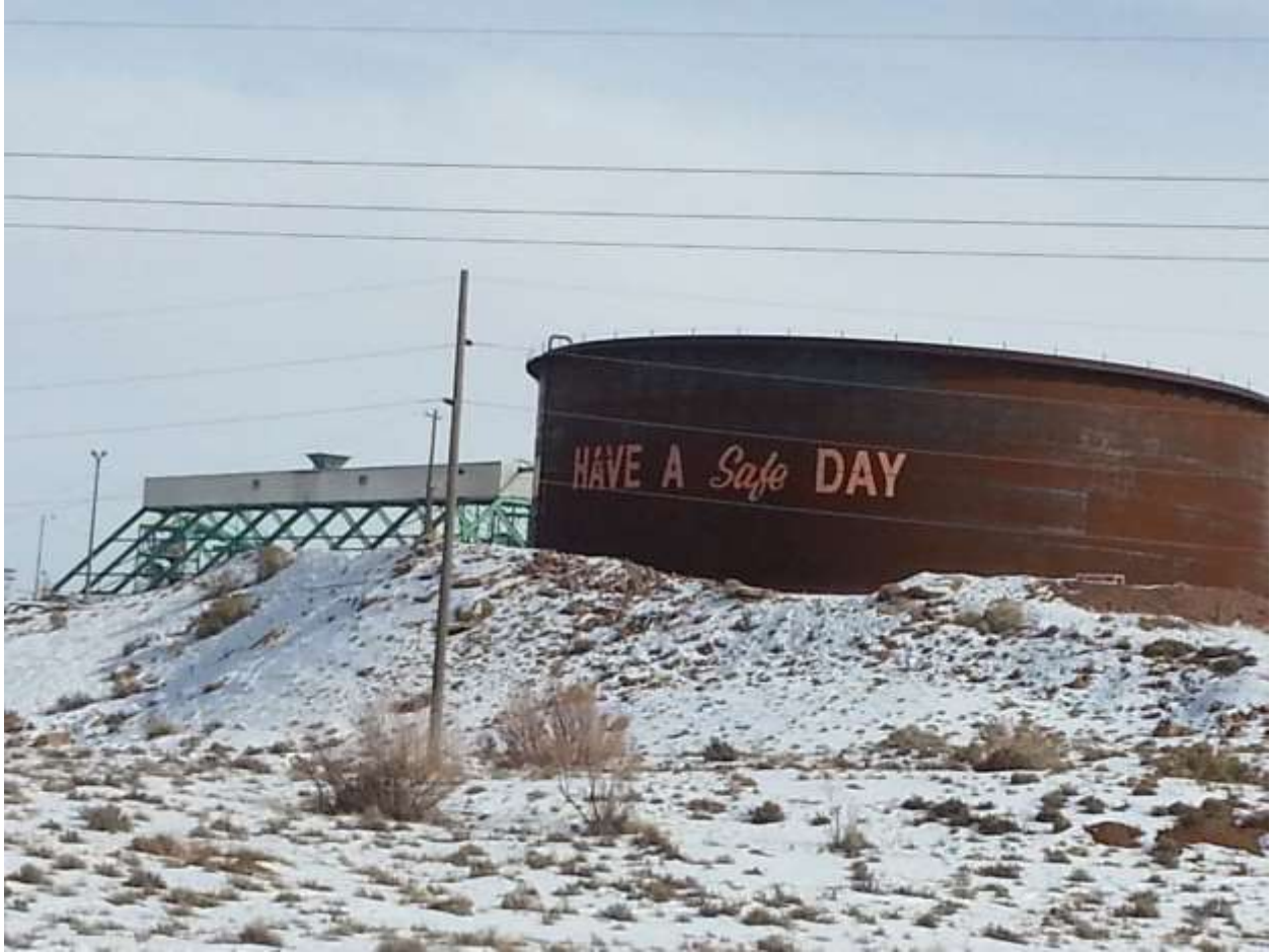
Figure 9: Coal Slurry Tank Next to Fenceline Home
