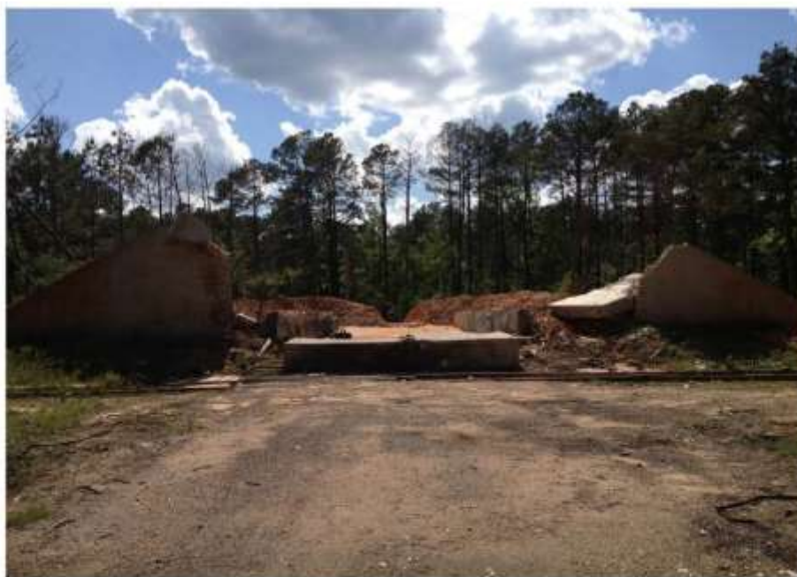
Photo 3: Result of explosion of magazine storing black powder and tractor trailers storing M6 Propellant in October 2012
