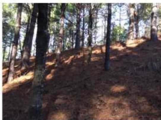
Photo 5: Trees growing on top of explosive storage magazine at Camp Minden
