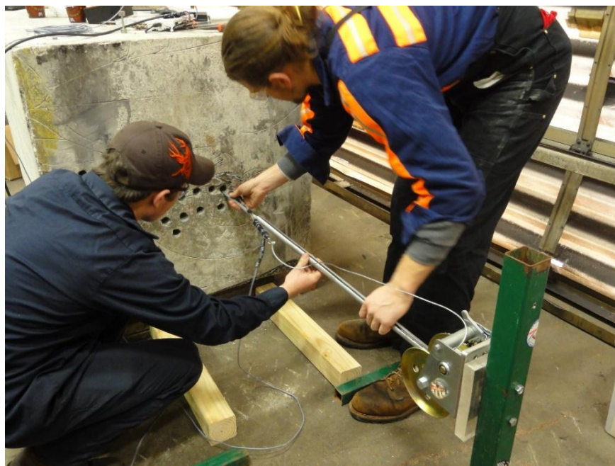
Figure 4.1: Installation of the Scratcher into the Borehole
