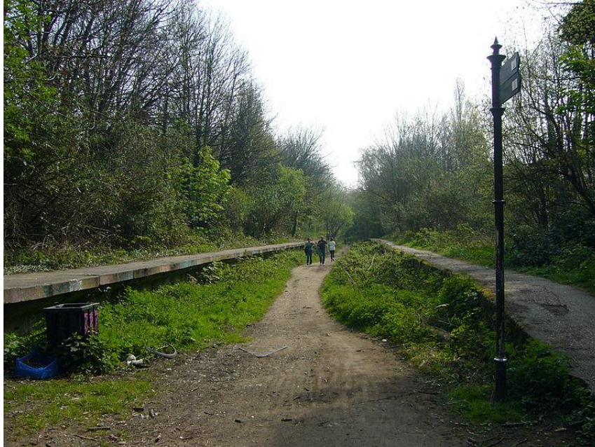
Figure 4.15 Railway Platforms on Parkland Walk, London, UK (Source : Fezpp 2007
