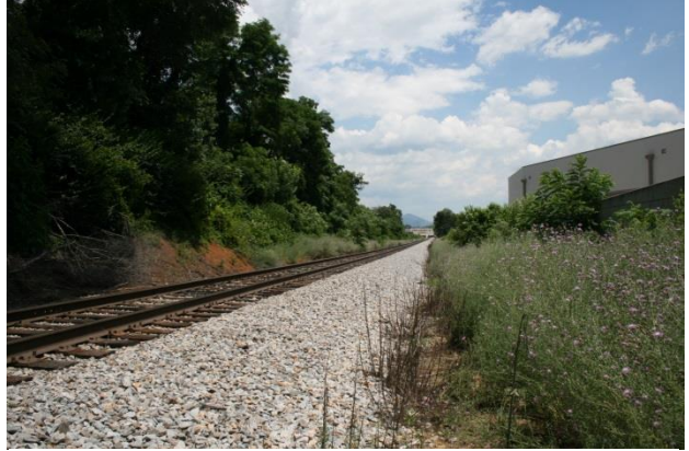
Figure 4.10 Wild vegetation growing along the railroad tracks, City of Roanoke, Virginia
