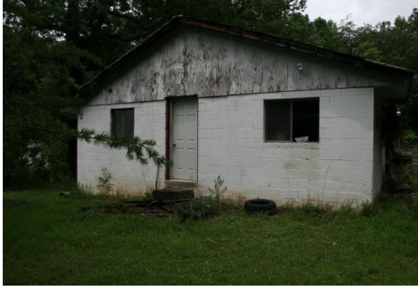
Figure 4.3 Derelict residential building, City of Roanoke, Virginia
