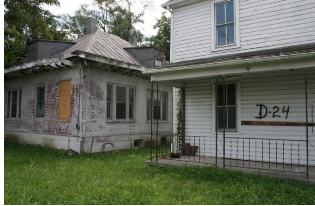
Figure 4.4 Two adjacent derelict residential buildings, City of Roanoke, Virginia
