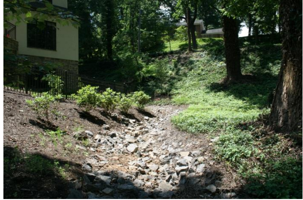
Figure 4.8 Residential drainage, City of Roanoke, Virginia
