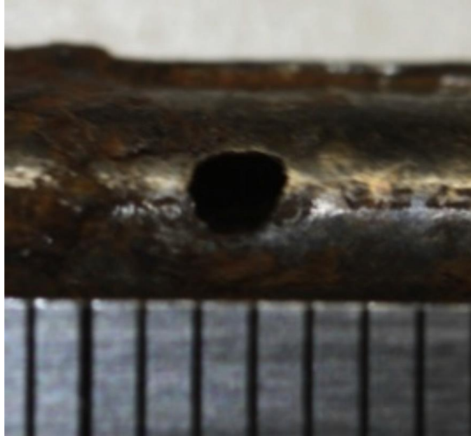
Figure 1-7: Pitting corrosion in chloraminated system.
