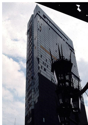
Figure 1.1 Wind induced vibration causes the fall of window glass on Hancock Tower [2]
