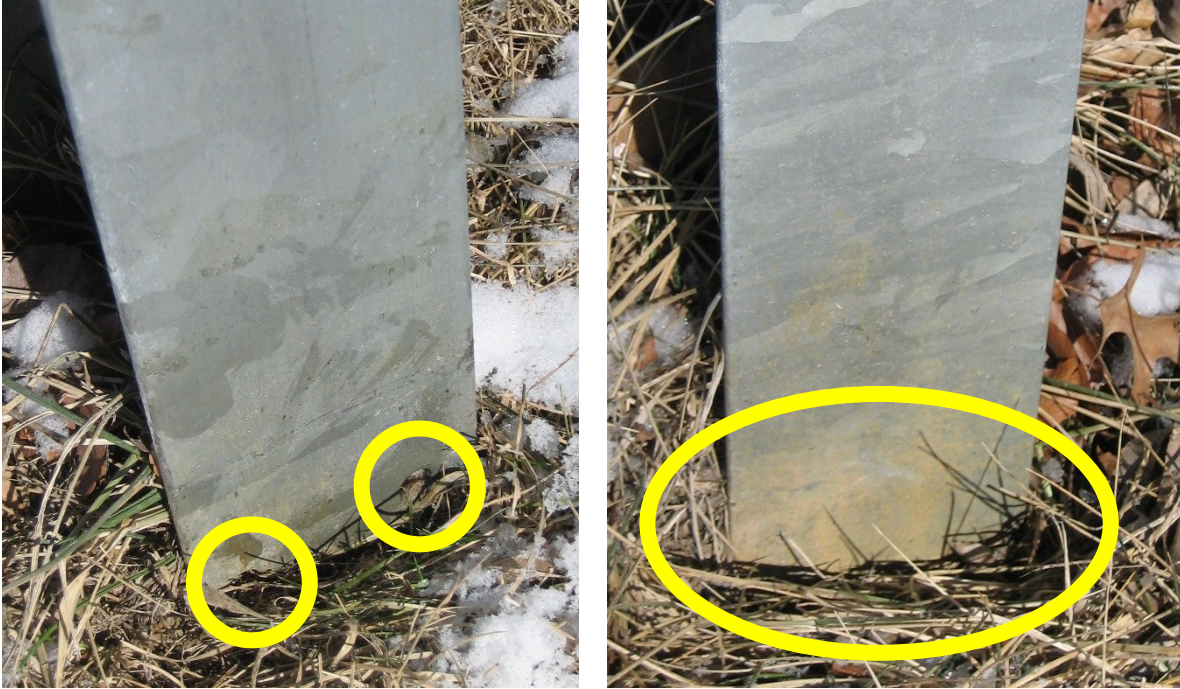
Figure A.8. It is a simple matter to distinguish the SYTP from standard non-breakaway steel posts, but in the field, it frequently requires careful, close observation. The distinguishing holes of the SYTP may be obscured by vegetation, or may be slightly below ground level.
