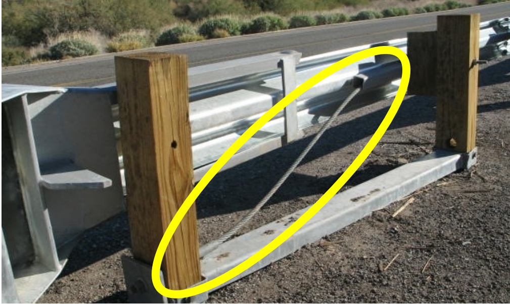
Figure A.4. Most, but not all, end terminal systems use anchor cables connecting the bottom of the first post to the top of the second post to help maintain tension in the guardrail.
