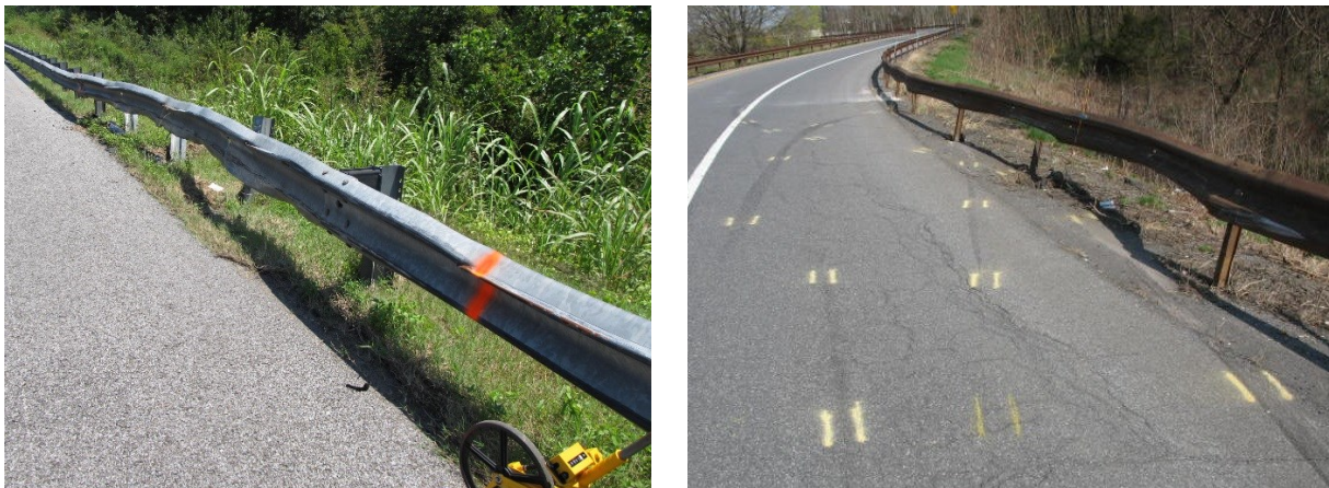
Figure 1.4. Left: damaged strong-post W-beam guardrail. Right: damaged weak-post W-beam guardrail.
