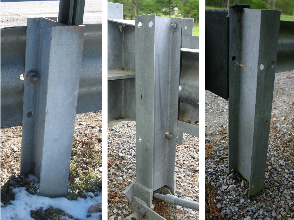
Figure A.7. Left: standard, non-breakaway steel post. Center: an example of a steel breakaway post with a typically conspicuous base design (in this example, a shearing-bolt design). Right: a Steel Yielding Terminal Post, or SYTP, is a breakaway steel post whose only distinguishing feature is four 1/2" holes drilled in the flanges at roughly ground level.
