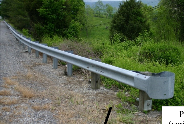
No Ground Strut, No Blockout On Post 2
