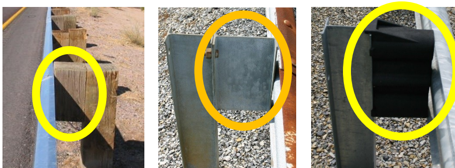
Figure A.9. Wood blockouts (left), steel blockouts (center) and composite blockouts (right).
