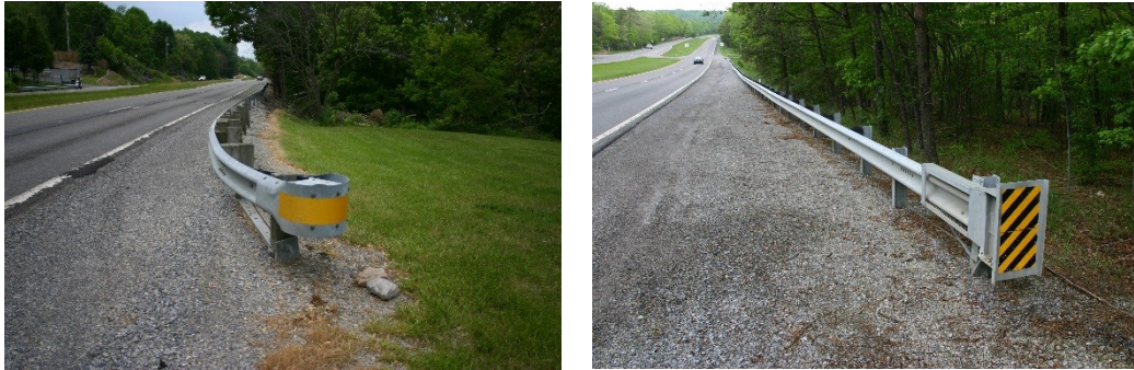
Figure A.2. Examples of non-energy-absorbing (left) and energy-absorbing (right) terminals.
