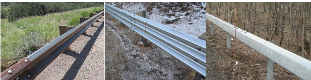
Figure 1.3. Common types of rail used in guardrail. From left: W-beam, thrie-beam, box-beam.
