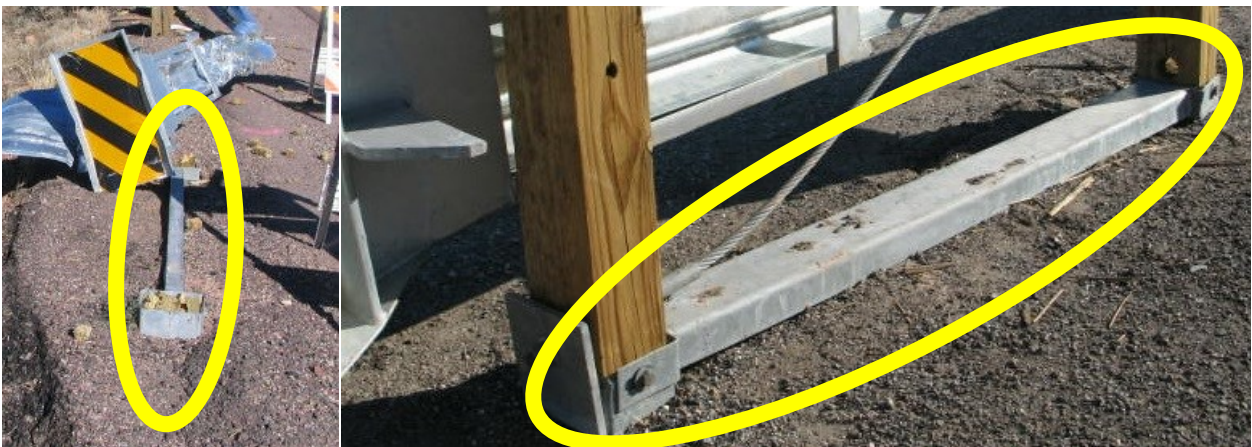
Figure A.5. Many end terminal system incorporate a ground strut, which is a beam connecting the first two posts in the system at ground level.
