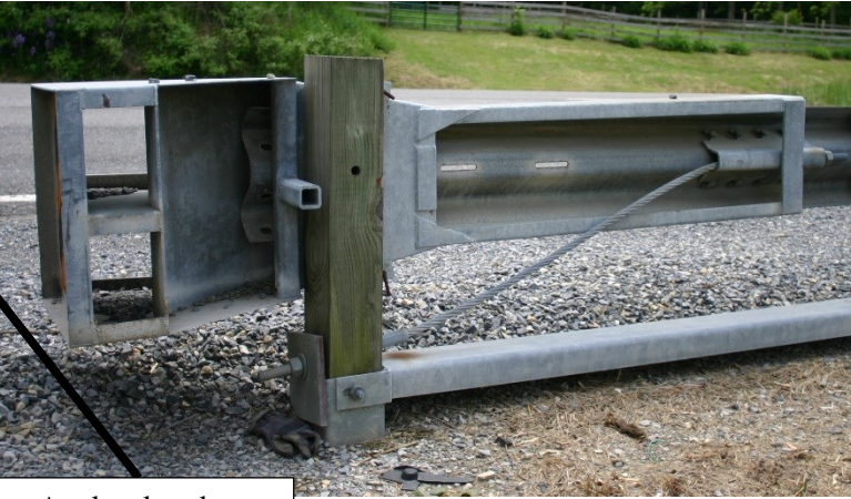
Anchor bracket hooks onto 8 bolts
