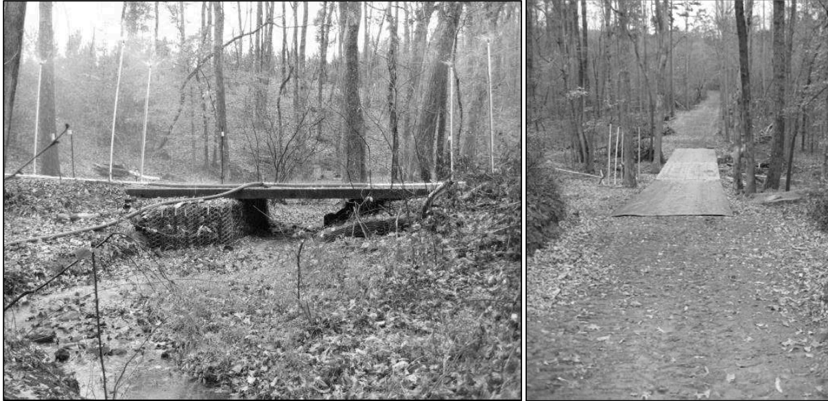
Figure 1: Left, bridge during rainfall simulation on BMP+ treatment with gabion basket as an abutment (left of stream) and the road running surface and bare soil rocked. Right, bridge prior to application of rock over the geo-textile on the running surface of the road (BMP), picture shows geo-textile prior to rock application which completed the BMP treatment, rock was applied over the geo-textile.
