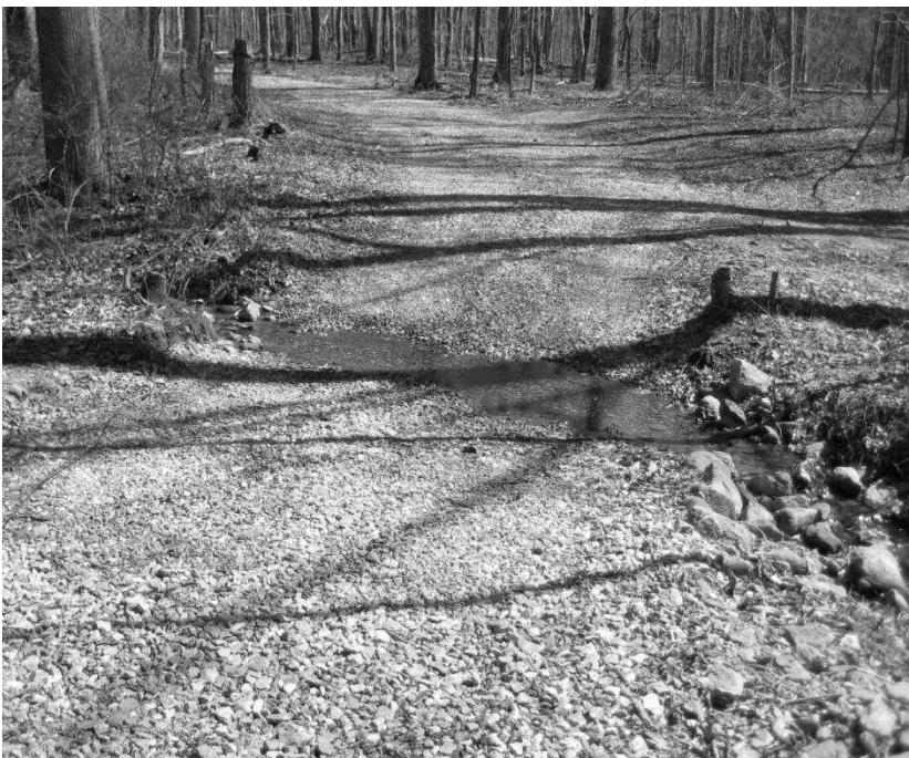
Figure 3: Ford crossing with BMP+ treatment including rocked running surface and Geo-Web in the channel.
