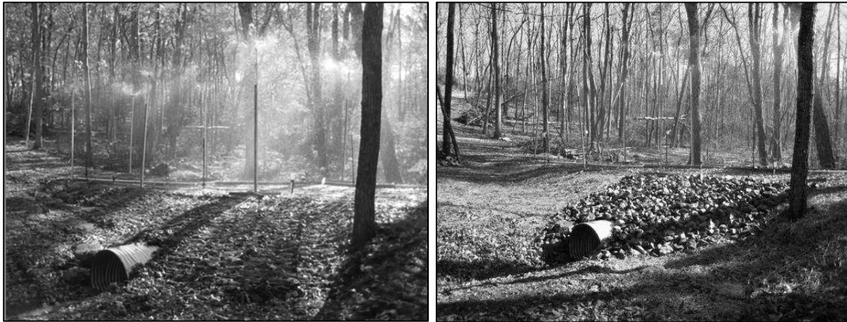
Figure 2: Culvert after installation and during BMP- rainfall simulation (Left), Culvert prior to BMP+ rainfall simulation with rocked running surface and fill slopes and seed and mulch on bare soil (Right).
