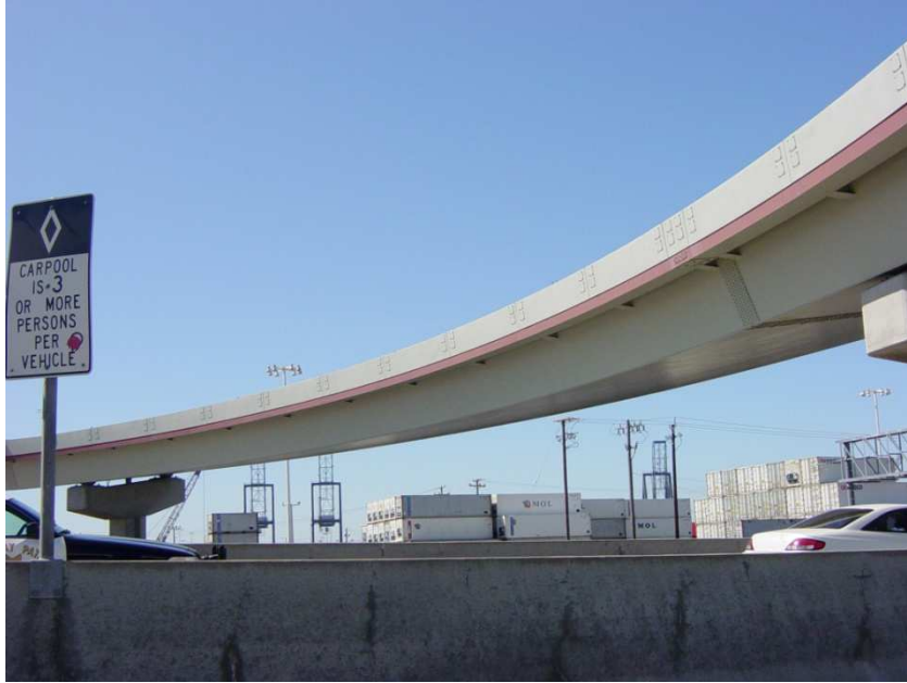
Figure 5-1: Highway bridge structure with tub girder (photograph from Leonard G.)
