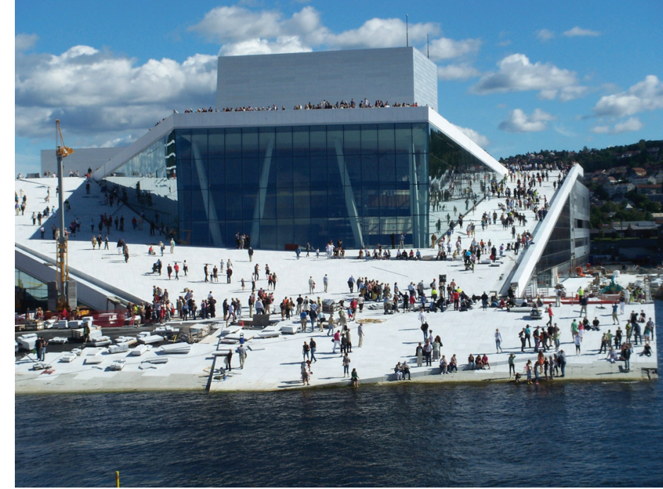
View of the accessible roof and the water's edge during construction
