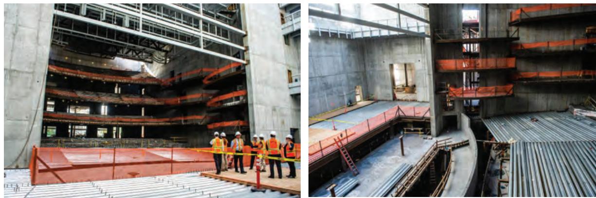
Photographs, Smart, Christopher. Construction of Salt Lake City's mega-theater.
