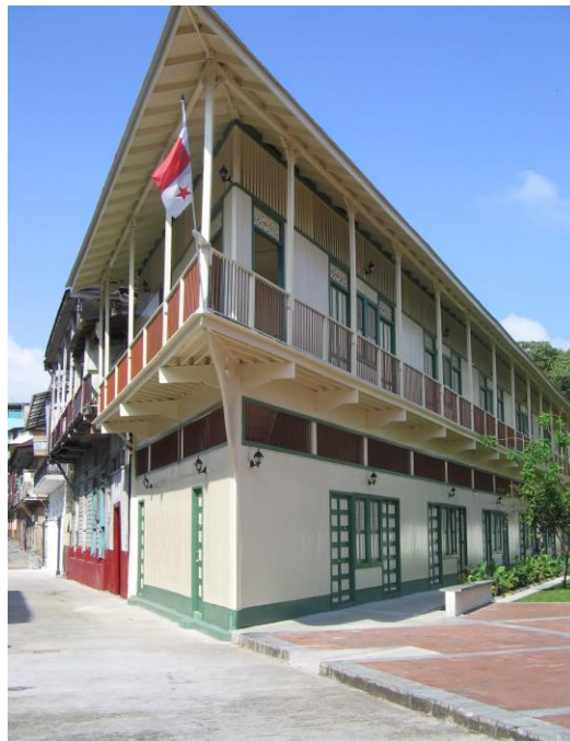
Figure 5.7. The Boyacá House Restored
