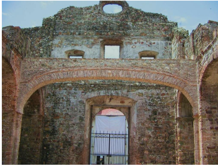
Figure 5.5. The Arco Chato Restored. April 10, 2007
