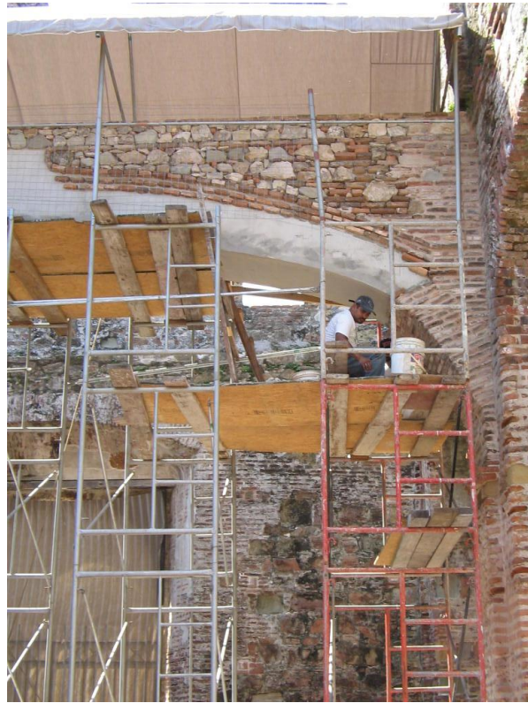
Figure 5.4. In the Process of Restoring the Chato Arch February 6, 2007
