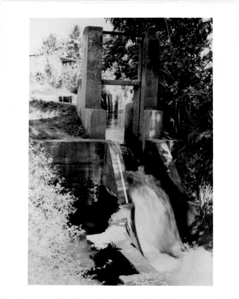
Plate 23. The same channel section as in plate 22. Note the result of patch work maintenance due to inadequate funds and supervision.
