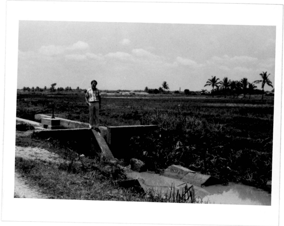
Plate 25. This picture was taken after the channel maintenance during 1984 Yala. Note the soil piled up on the left bank of the channel to fill up eroded bank.
