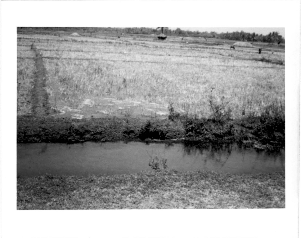
Plate 18. Same channel as in plate 17, a little further downstream. Encroachments have weakened the channel bund. A farmer obtained more water from large hole made in the channel bank.
