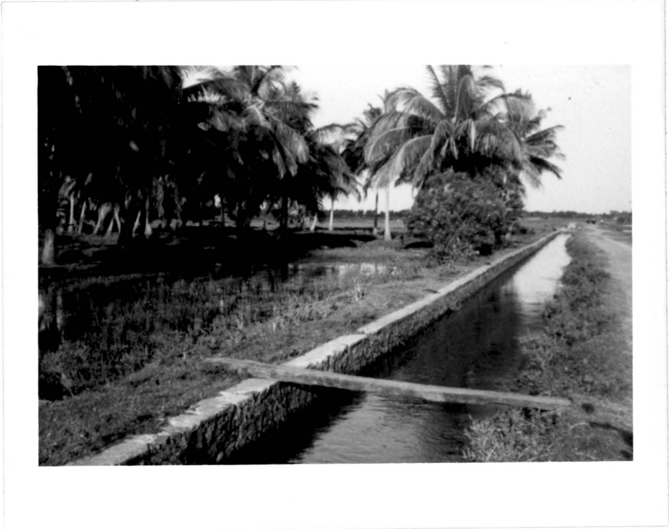
Plate 12. Upstream view of the distributory channel to tract 2. Note the water filled highland allotments cultivated to paddy. This land was cultivated during both seasons.
