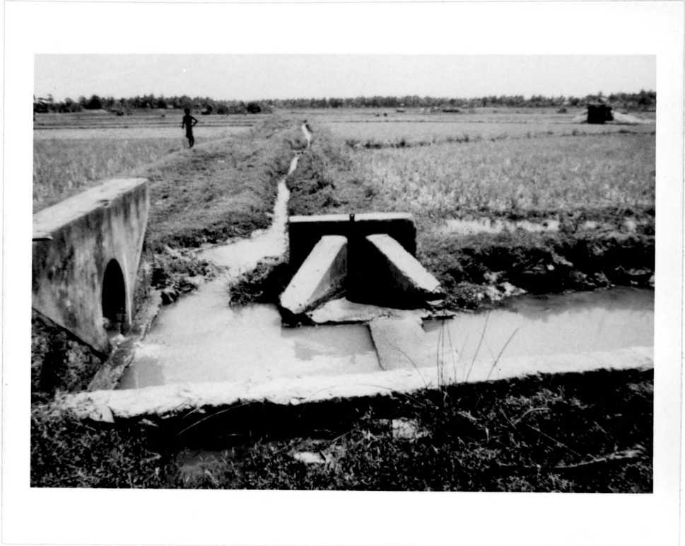
Plate 15. A midway along the distributory channel to tract 2. Note the defunct flow control structure. Water was directly obtained from the channel by opening the channel embankment. Thus, water control downstream has become impossible.
