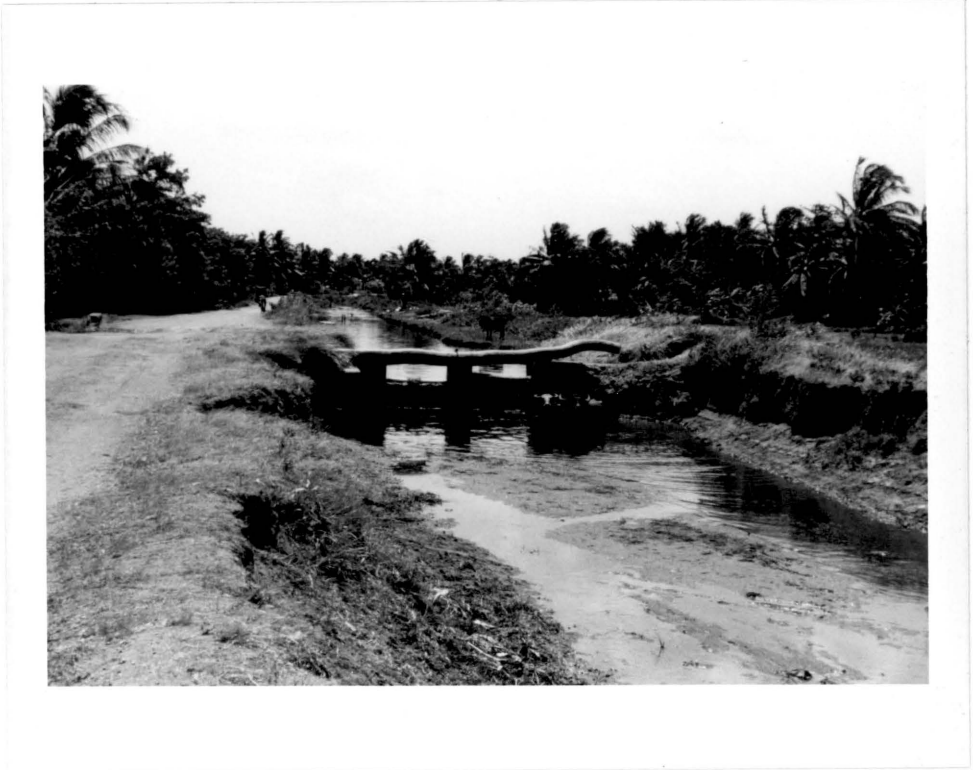
Plate 10. A view of the main channel at low flow. A temporary dam obstructs the flow below the log bridge. Notice the eroded banks of the channel.
