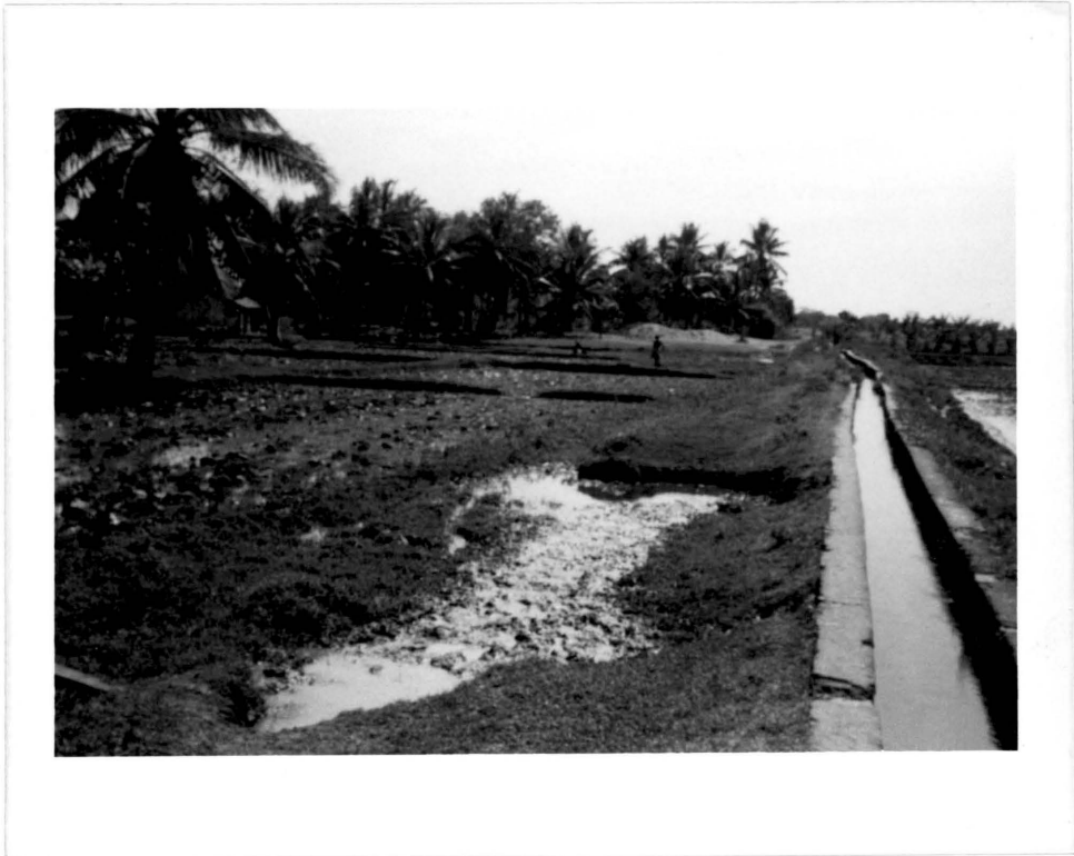
Plate 14. Same channel as in plate 13 but further down stream. The left bank supposed to serve as a road and the channel lining has been damaged to obtain water to the highland on the left.
