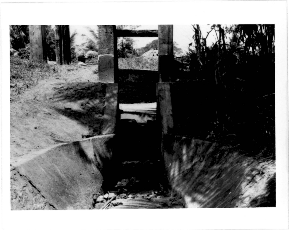
Plate 22. A down stream view of tract 8 distributory head work. The picture was taken soon after channel maintenance. Compare with plate 21 which was taken at the end of the season.
