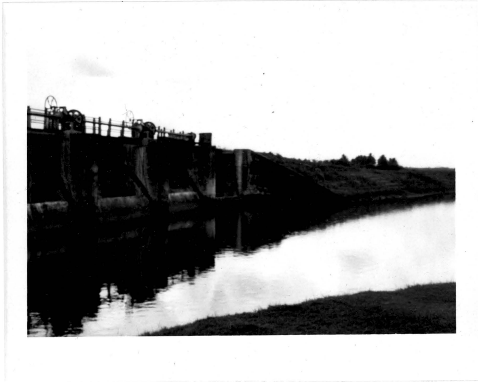
Plate 1. Kaudulla Oya Stage I anicut which diverts irrigation water into the main channel. The photograph was taken after the repair of flood damages during 1983 Maha season. The bund on the right was blasted to convey flood waters during the 1983 Maha because the radial gates could not be operated due to inadequate maintenance.
