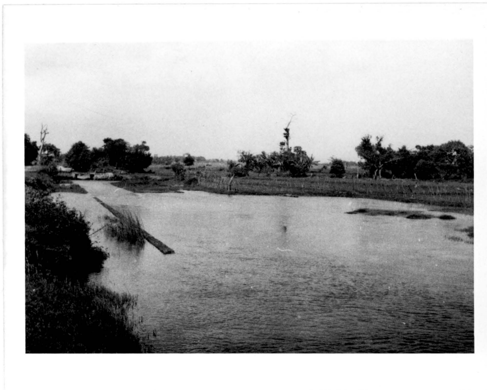
Plate 6. A downstream view of main channel from the tract 1 distributory offtake. The high velocity of flow caused by constriction at the overpass bridge and inadequate downstream bank protection at the transition has eroded and widened the channel.
