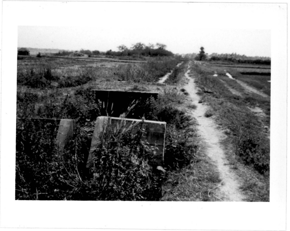
Plate 36. A defunct drop structure. The rule of thumb used by the Department of Irrigation is to constrict the channel to half the bottom width. This done to build sufficient head for pipe outlets immediately upstream. However, during heavy rains the flow in the channel overtops the bank thus, eroding the banks and finally leaving the structure in the middle.
