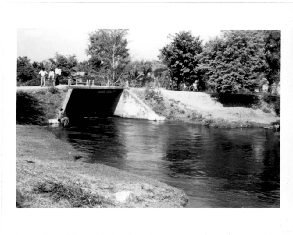
Plate 2. Overpass bridge and the flow control structure at the head of Kaudulla stage I main channel. Note the width of the channel in relation to bridge and the flooded embankments. The woman stands on the lined top of the channel.
