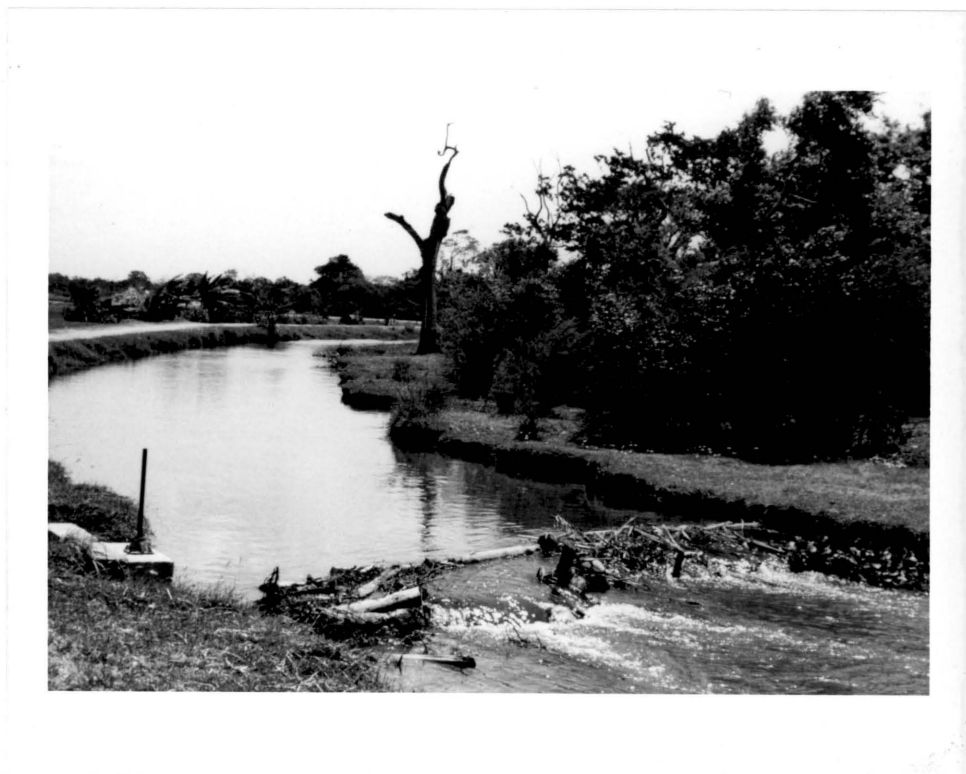
Plate 11. A temporary dam constructed by farmers across the main channel to build sufficient head for the distributory offtake.
