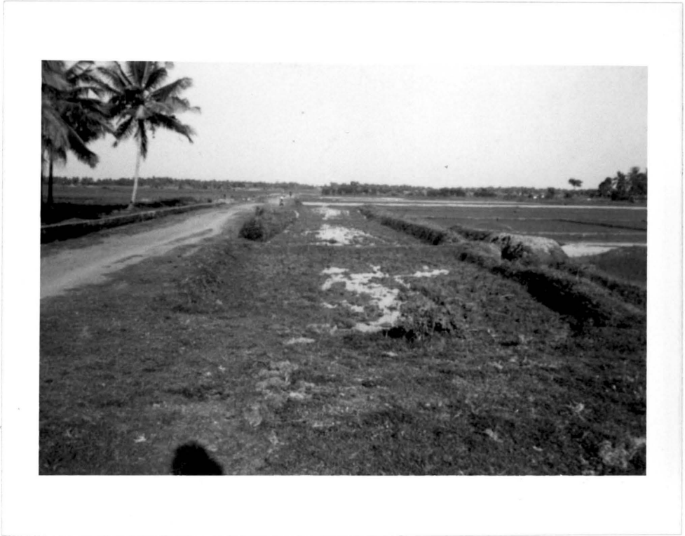
Plate 16. The road reservation encroached and converted to a paddy field in tract 2.
