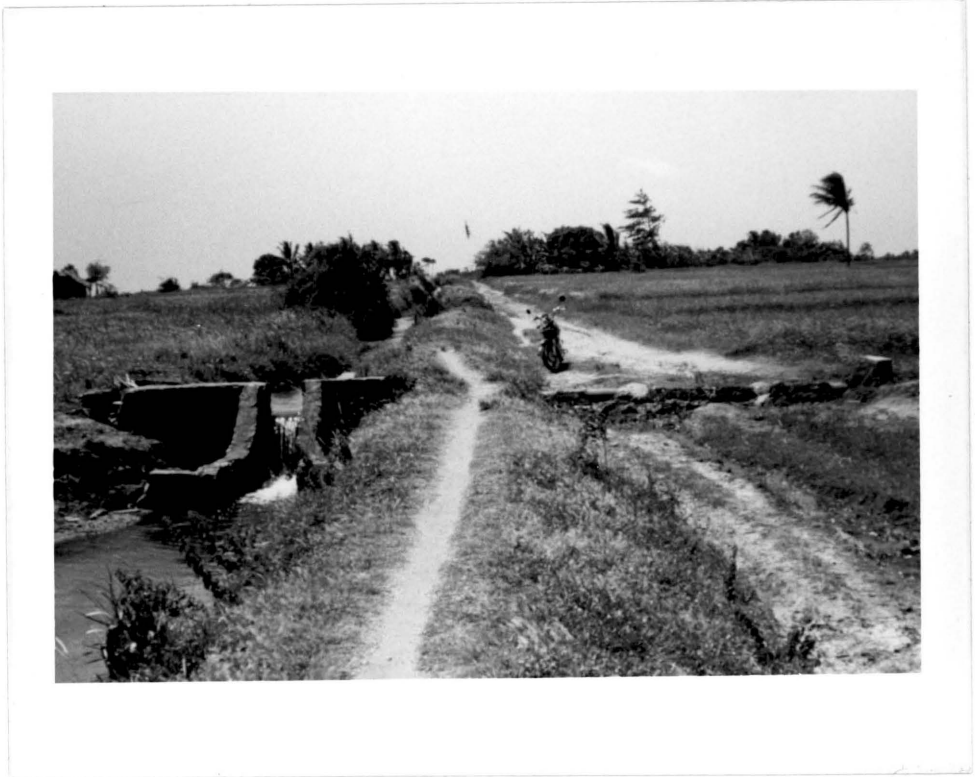
Plate 28. This is another picture of the tract 8 distributory about midway. The water from damaged pipe outlet laid across the road and distributory channel bank was conveyed along the road to the fields on the opposite side.
