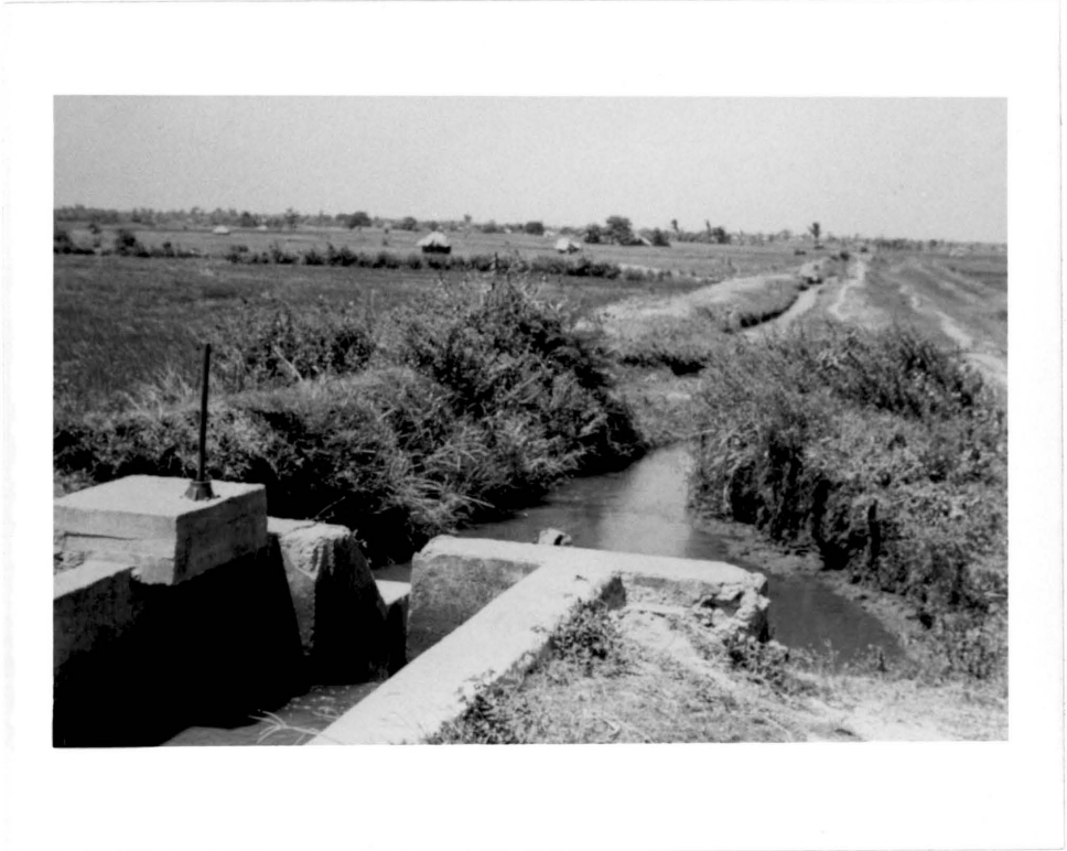
Plate 29. A drop structure in the tract 8 distributary. Note the erosion of the channel bank below the drop. The huts seen on the foreground are used by farmers to keep night watch in order to obtain their water supply.
