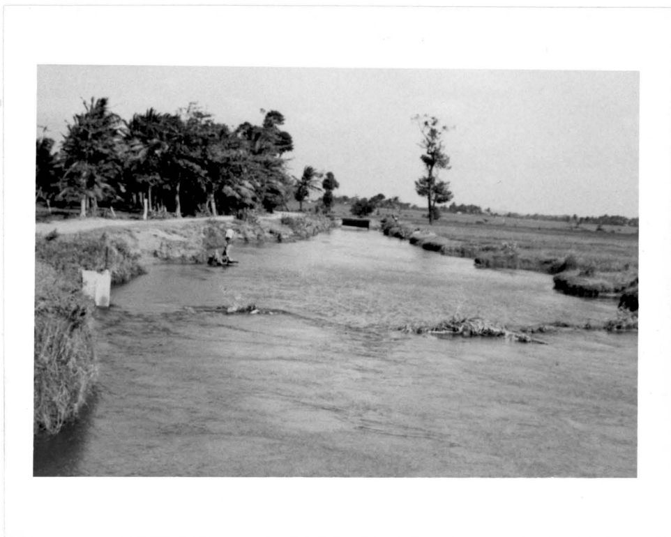
Plate 3. Main channel of stage I at the first field channel offtake. A view from down stream. On the right are the stage II irrigated fields. These fields release large amounts of drainage water into the main channel through numerous openings cut into the channel embankment. Note the width of the channel due to erosion and the attempt by farmers to head up water by piling up obstructions in the middle.
