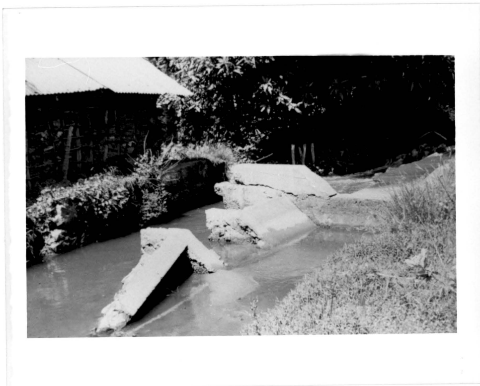
Plate 24. Same channel as in plate 22 about 20 meters down stream. The channel lining and weir type flow regulator have fallen apart. The water actually flowed over the compound of the hut in the background before getting into the channel at a point down stream.
