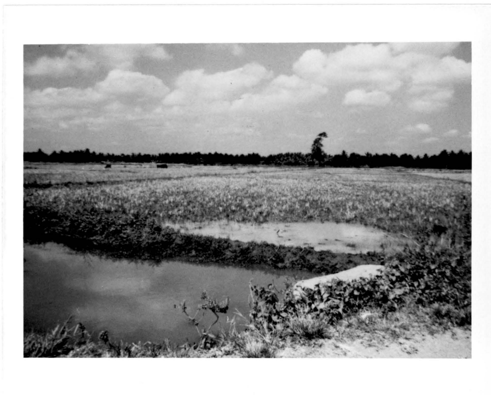
Plate 17. A view of the head reach of distributory channel 4. This is a relatively narrow and long distributory. The discharge from the main channel has considerably eroded the sides forming a large pool. The farm on the right has encroached the channel bank leaving hardly anything for the channel bank.
