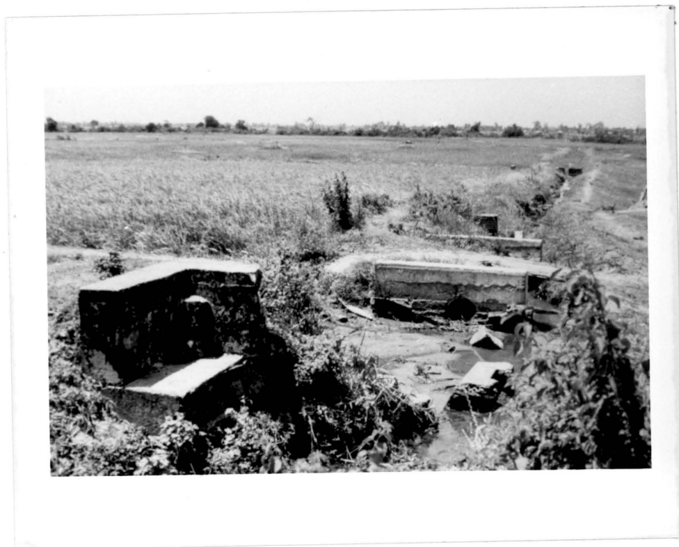
Plate 30. Tail end view of the tract 8 distributory channel. Water distribution was chaotic in this section of the channel. Note the structure on the left which was a defunct field channel offtake. Since channel water level was at a much lower level than the offtake the farmers served by this channel had to rely on water draining from the upstream fields.
