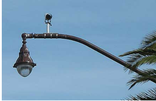
Figure 3.1: Traffic monitoring sensor installed on a light pole
