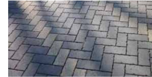
Permeable Unit Pavers
