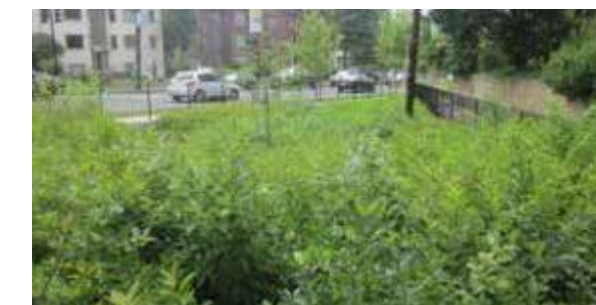
Bioretention in Open Area
