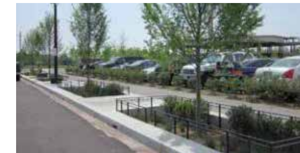
Bioretention Planter Adjacent to Roadway
