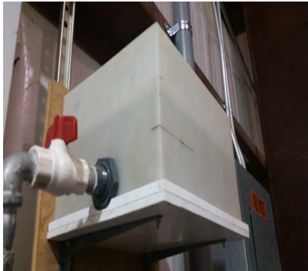
Figure B.3: Expansion tank of the ice making system.
