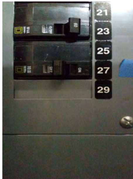
Figure B.2: Breaker switch for chiller system.
