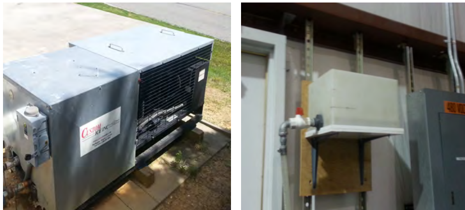
Figure 3.5: Left-Outdoor chiller unit of Terramechnaics Rig. Right-Ethylene glycol expansion tank.
