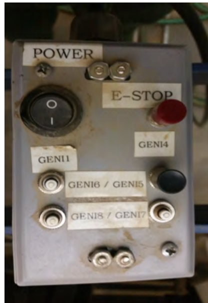
Figure A.2: Emergency Stop switch on controller of the Terramechanics Rig
