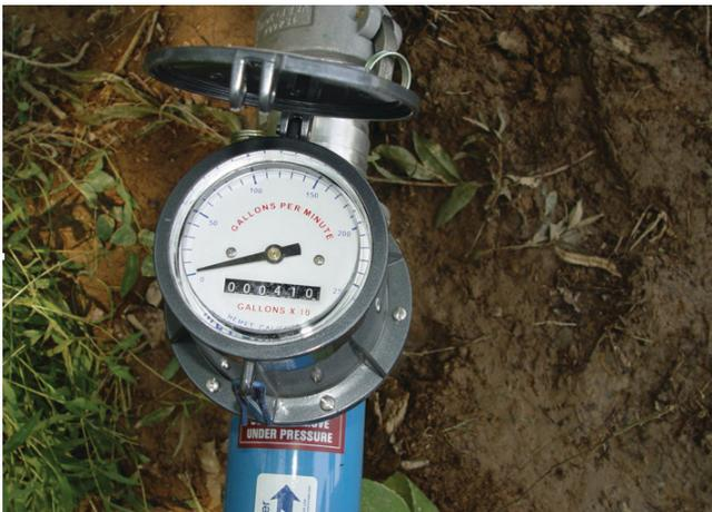
Figure 8. Flow meter for measuring the volume of water through pipes. (Photo: Anthony LeBude)
