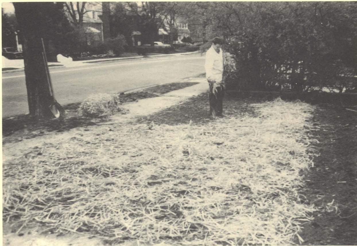
Figure 7. Straw mulch being hand applied at 1.5 bales per 1,000 square feet to a newly seeded area.
