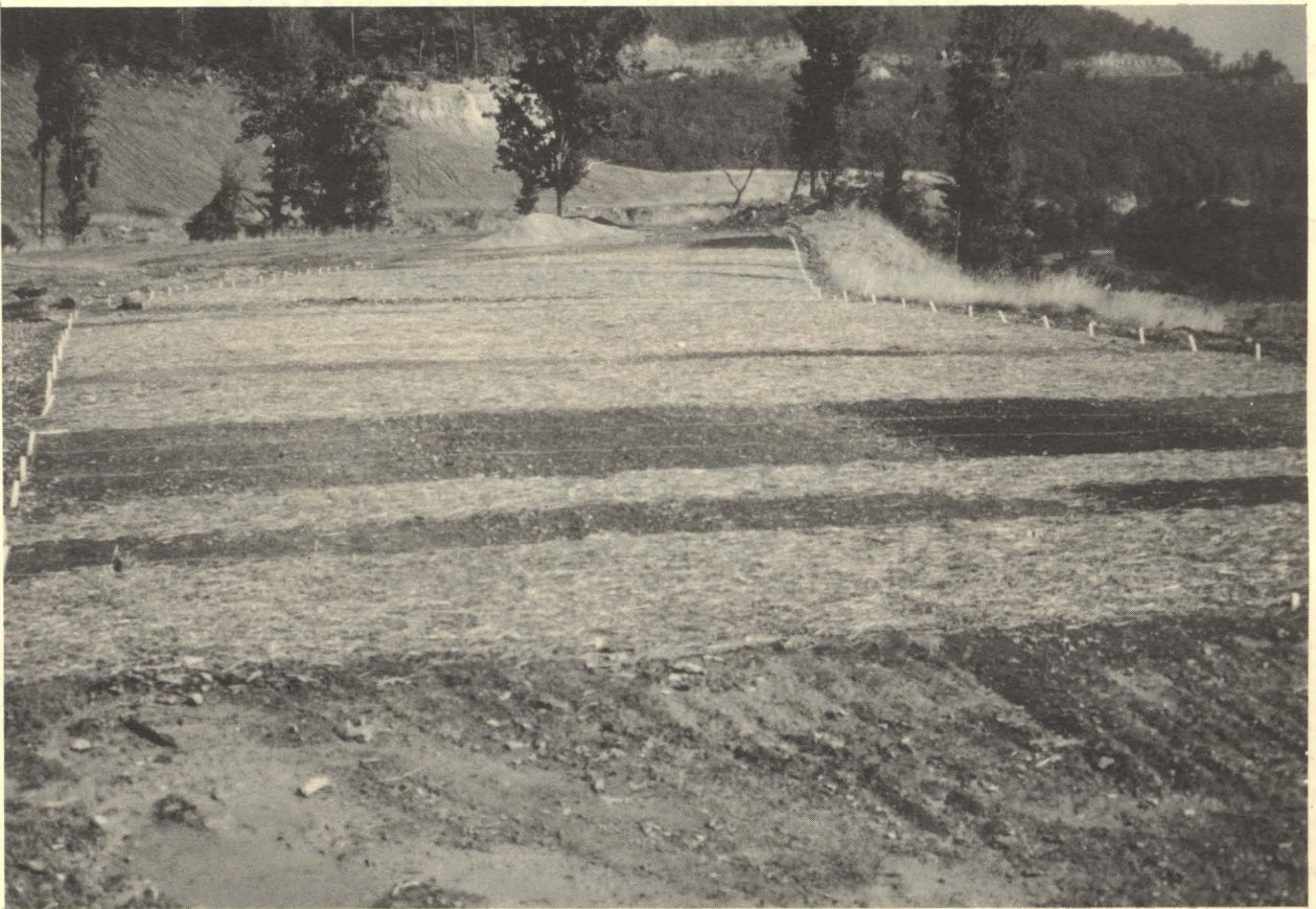
Figure 1. Sodding, seeding and sprigging methods were evaluated on 20 different turfgrass types grown on unamended mine soil, and mine soil amended with sawdust, topsoil and composted sludge. This picture was taken in September 1980, shortly after establishment.
