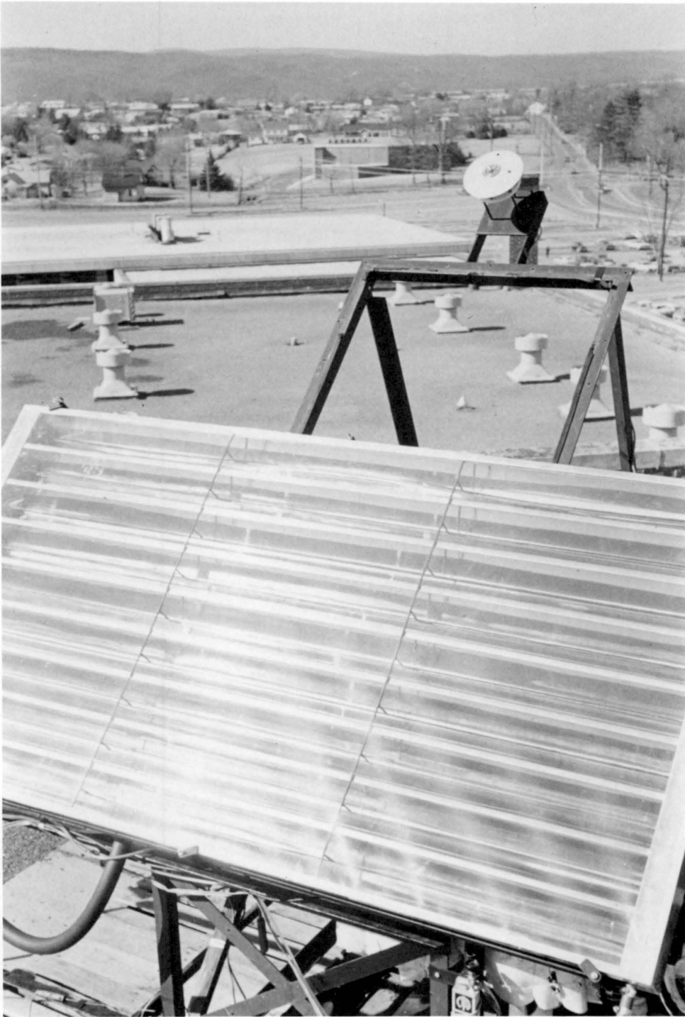
Fig. 3. Cylindrical Parabolic Solar Collector Manufactured by Martin Processing Co., Inc.
