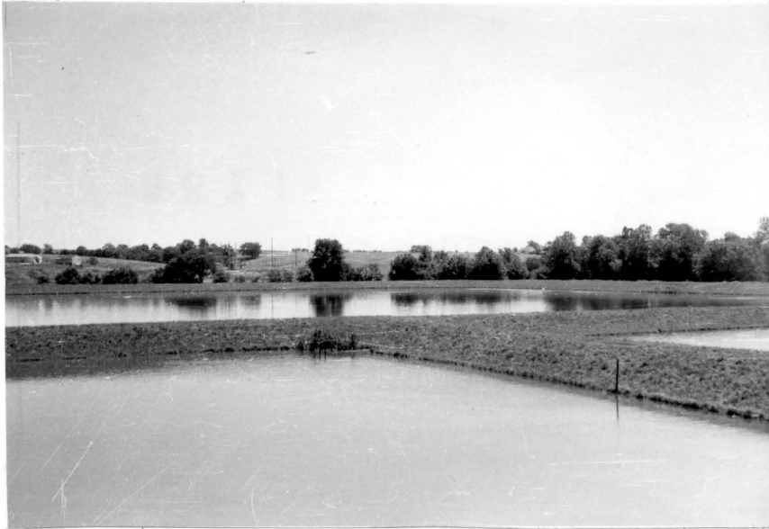
1. VIEW ACROSS THE WIDTH OF THE FAYETTE SEWAGE LAGOON SYSTEM.
