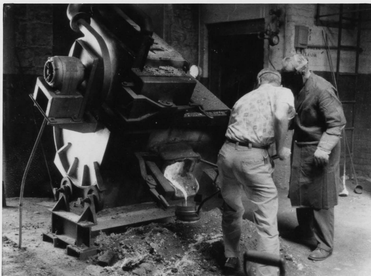
Tapping of Metal from Furnace
